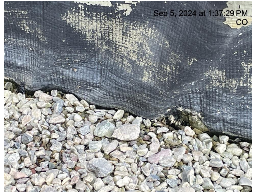
Photo # 8322 Hole in liner/liner needs maintenance
