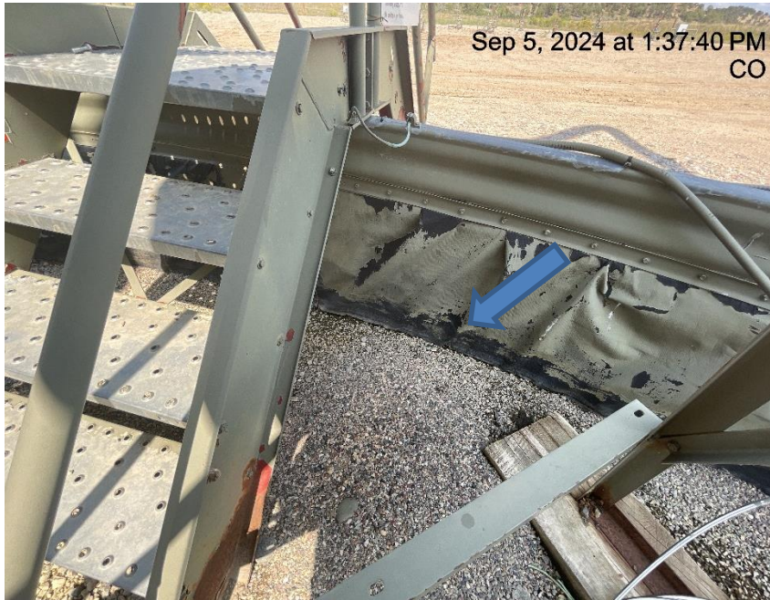
Photo # 8321 Hole in liner/liner needs maintenance
