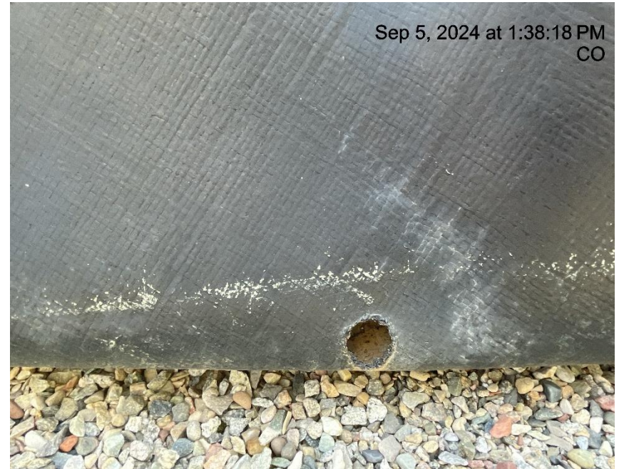
Photo # 8326 Hole in liner/liner needs maintenance
