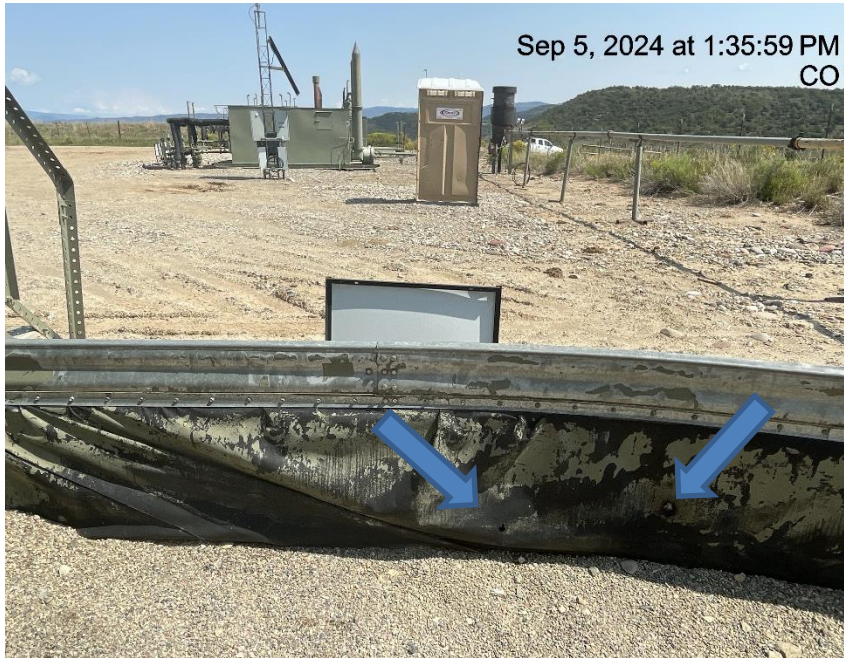
Photo # 8317 Multiple holes in liner/liner needs maintenance
