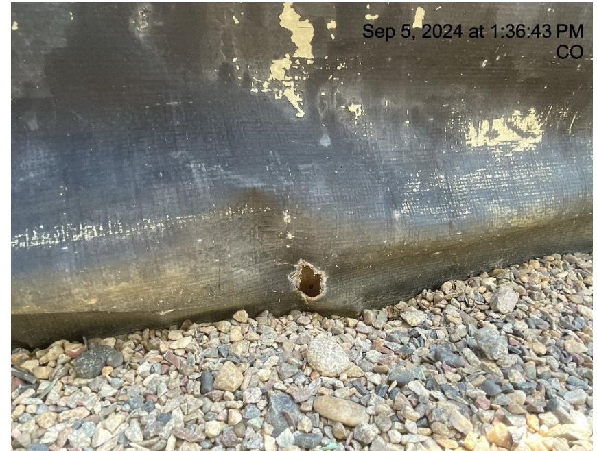
Photo # 8320 Hole in liner/liner needs maintenance
