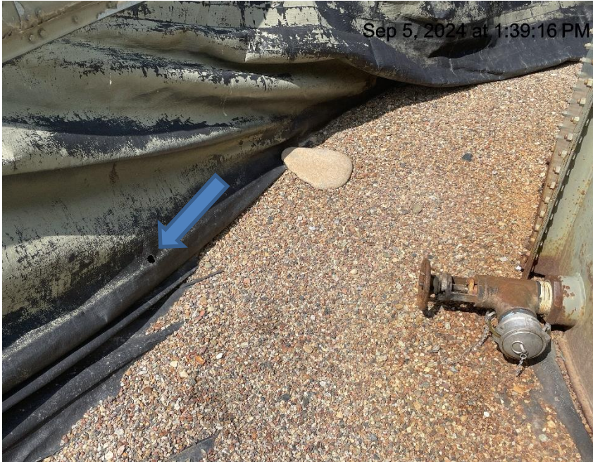
Photo # 8329 Hole in liner/liner needs maintenance
