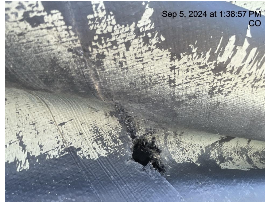
Photo # 8328 Hole in liner/liner needs maintenance
