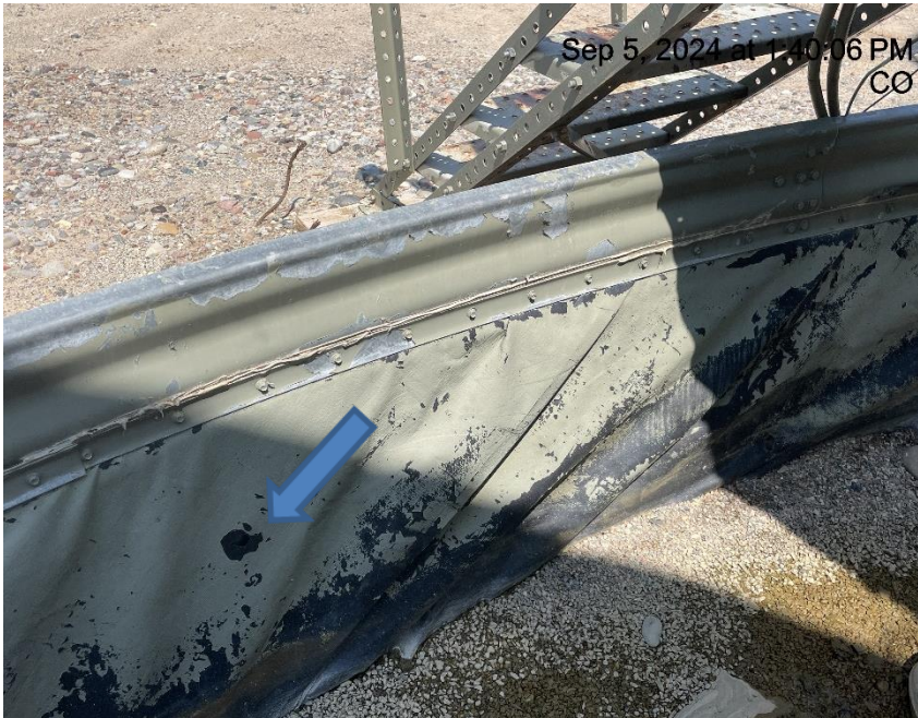
Photo # 8331 Hole in liner/liner needs maintenance
