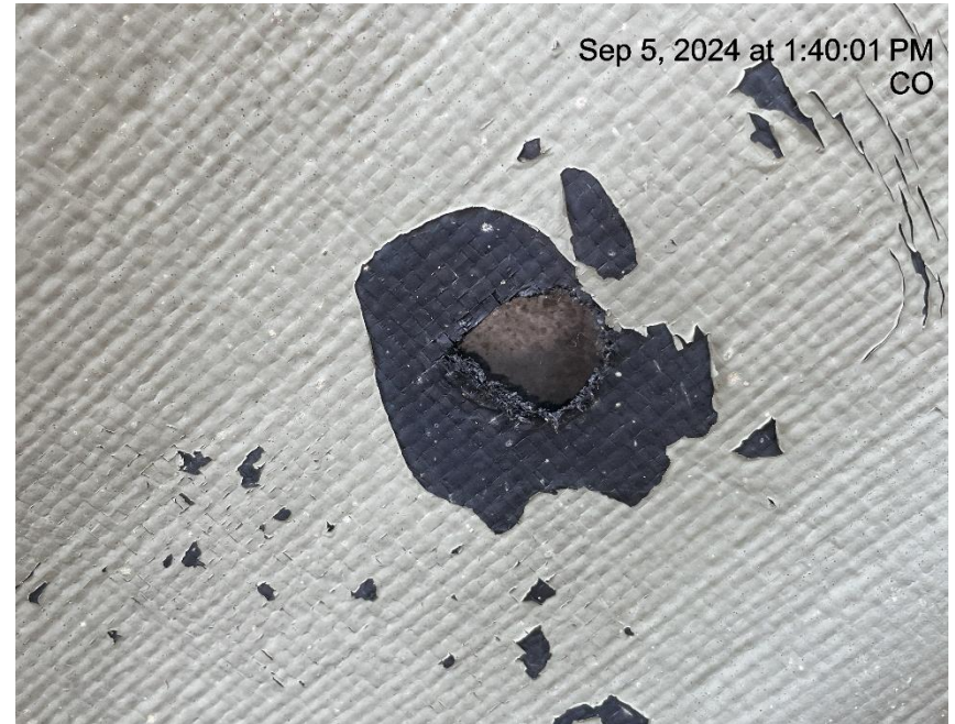
Photo # 8332 Hole in liner/liner needs maintenance
