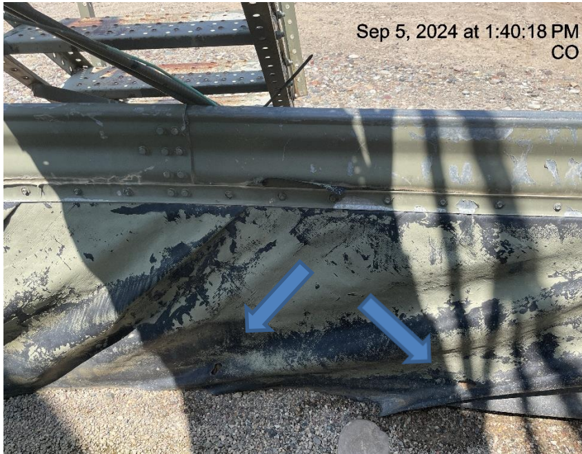
Photo # 8333 Multiple holes in liner/liner needs maintenance
