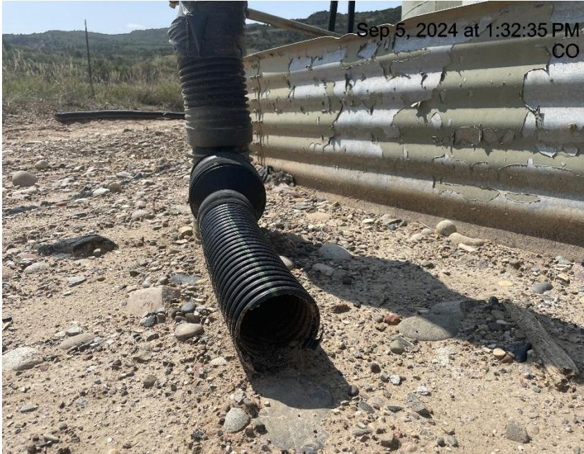
Photo # 8343 Flowline heating insulation open ended /available for entry by wildlife/wildlife hazard
