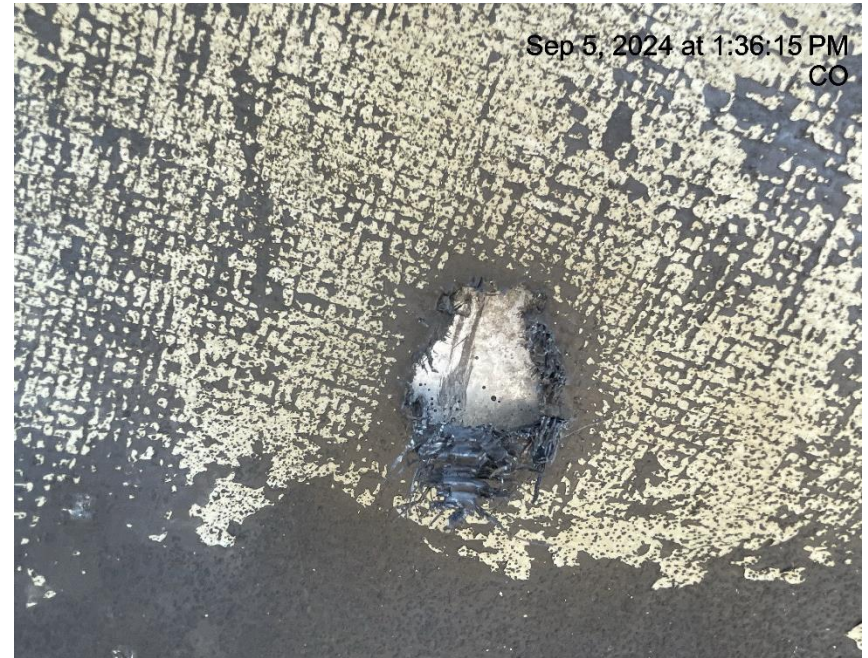
Photo # 8318 Hole in liner/liner needs maintenance
