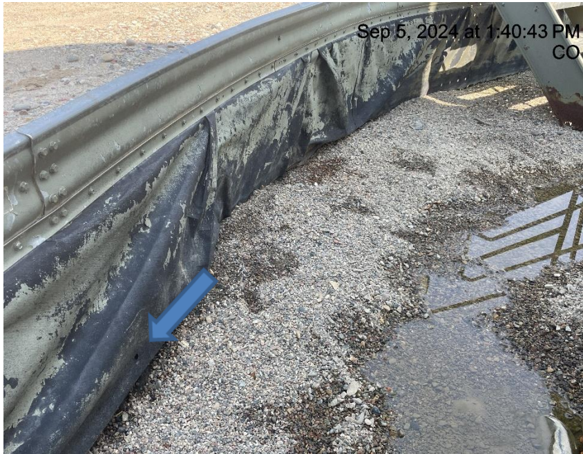
Photo # 8337 Hole in liner/liner needs maintenance
