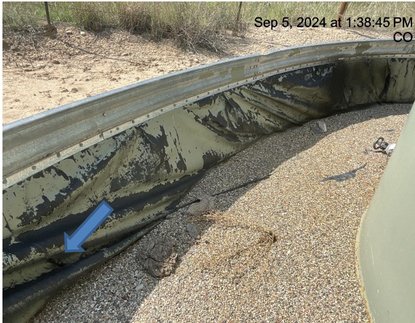
Photo # 8327 Hole in liner/liner needs maintenance
