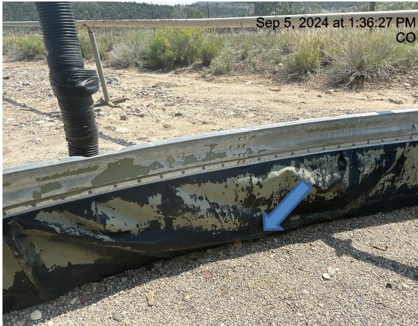
Photo # 8319 Hole in liner/liner needs maintenance
