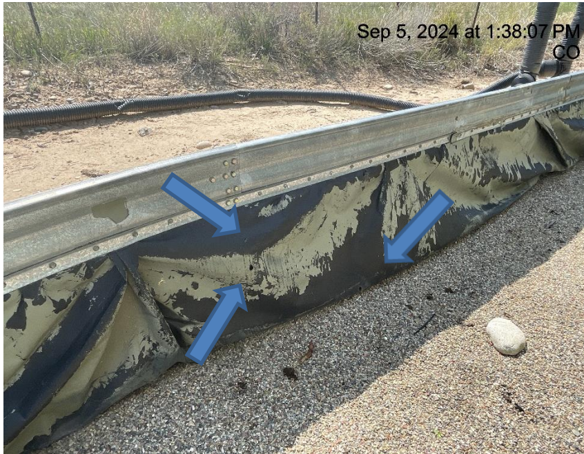
Photo # 8323 Multiple holes in liner/liner needs maintenance
