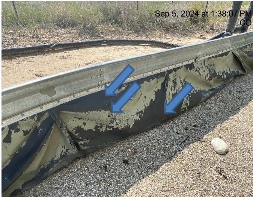
Photo # 8325 Multiple holes in liner/liner needs maintenance
