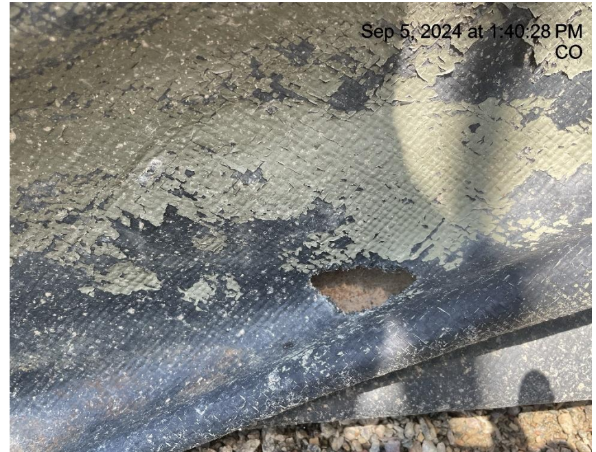
Photo # 8336 Hole in liner/liner needs maintenance
