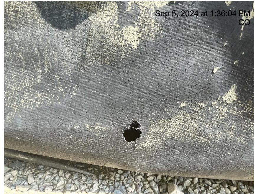
Photo # 8316 Hole in liner/liner needs maintenance
