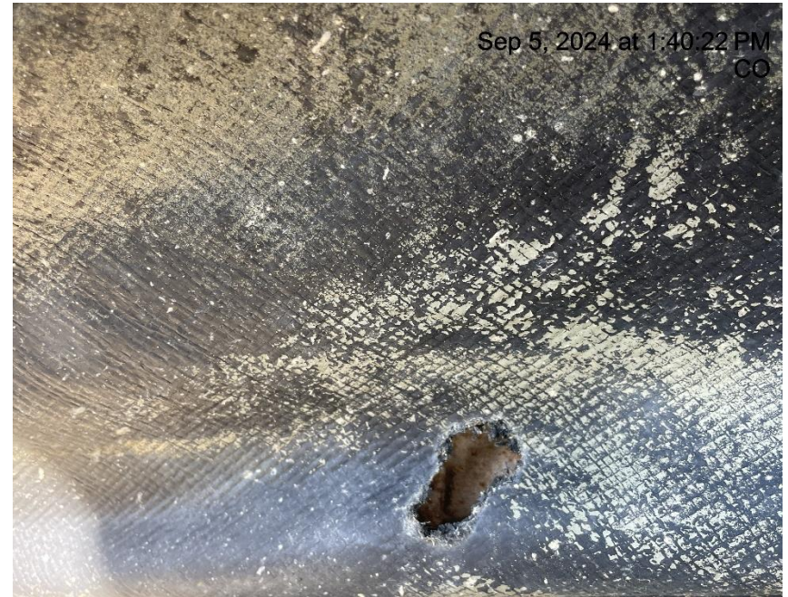
Photo # 8334 Hole in liner/liner needs maintenance
