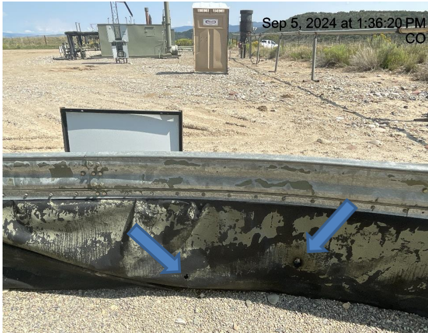
Photo # 8315 Multiple holes in liner/liner needs maintenance
