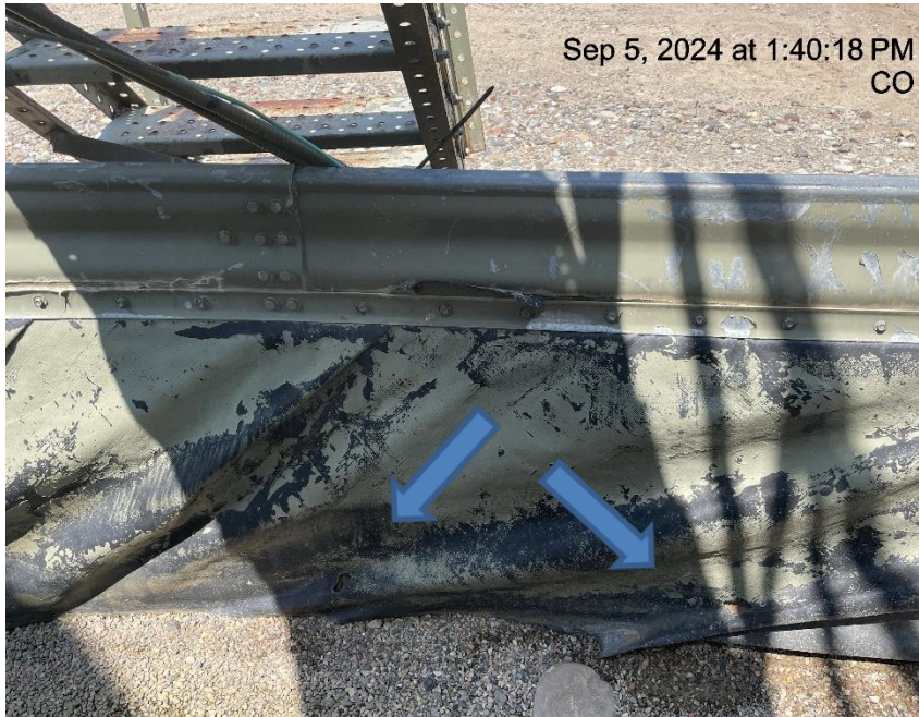
Photo # 8335 Multiple holes in liner/liner needs maintenance
