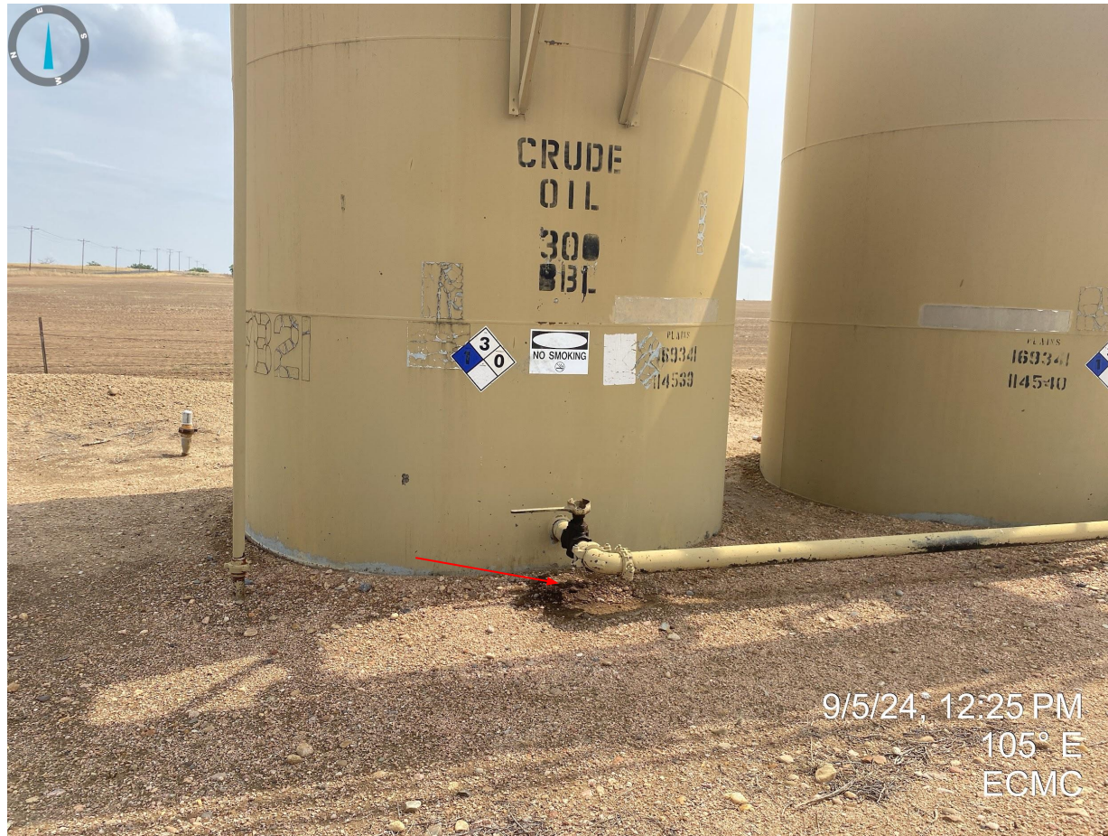
Photo 10. Stained soil observed near the northern vertical AST.
