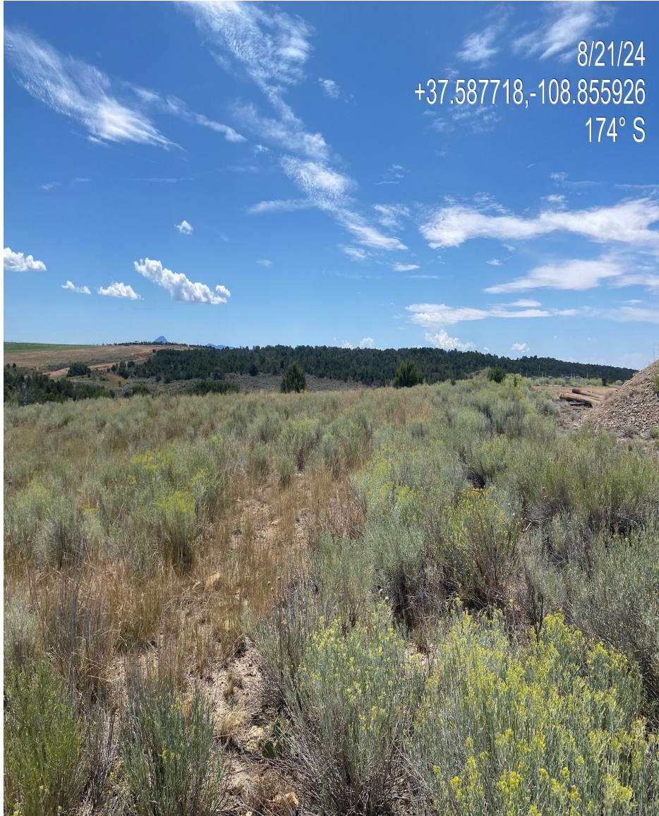
Photo 2. View of cut and fill slopes on location that are vegetated to ECMC's 80% of reference area standard.
