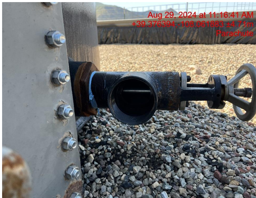
Open ended load line - Photo #05225
