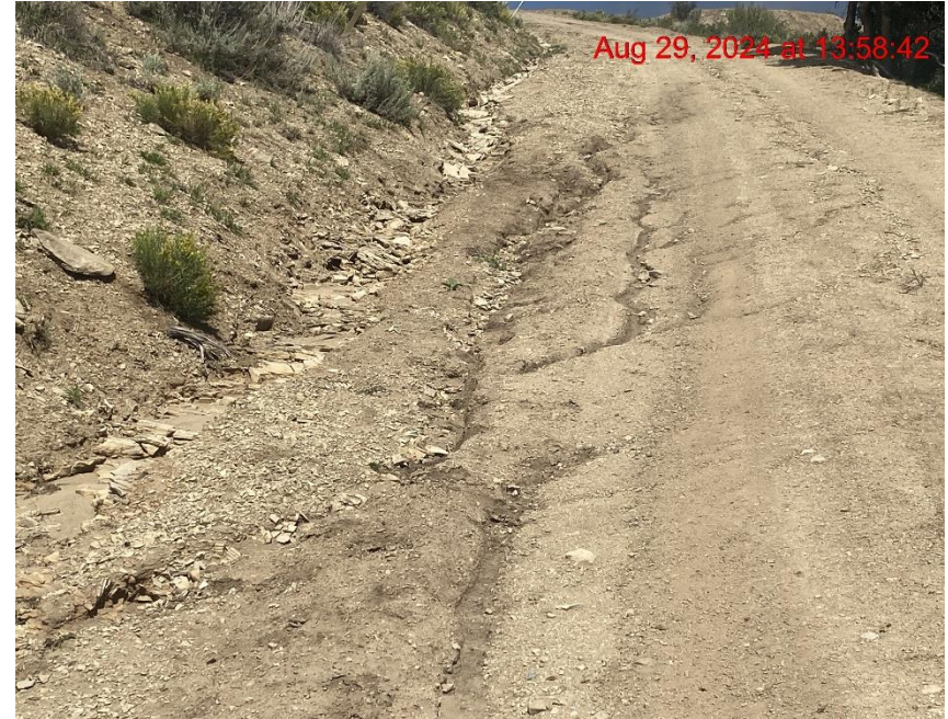
Insufficient Erosion Control – Photo #03211
