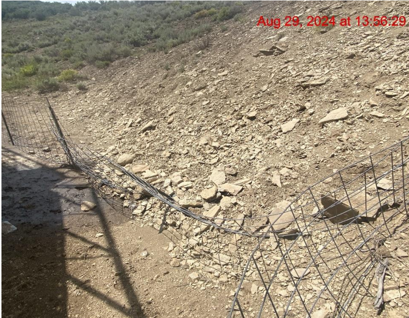
Insufficient Erosion Control/Damaged Fencing – Photo #03207
