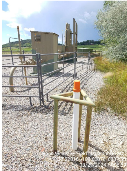
5. Cathodic protection riser on east side of meter shed
