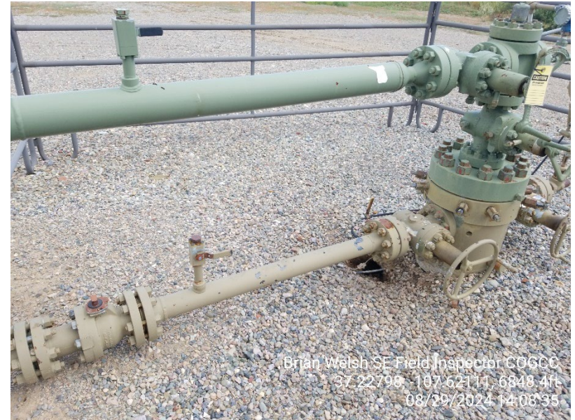
4. Casing valve SI
