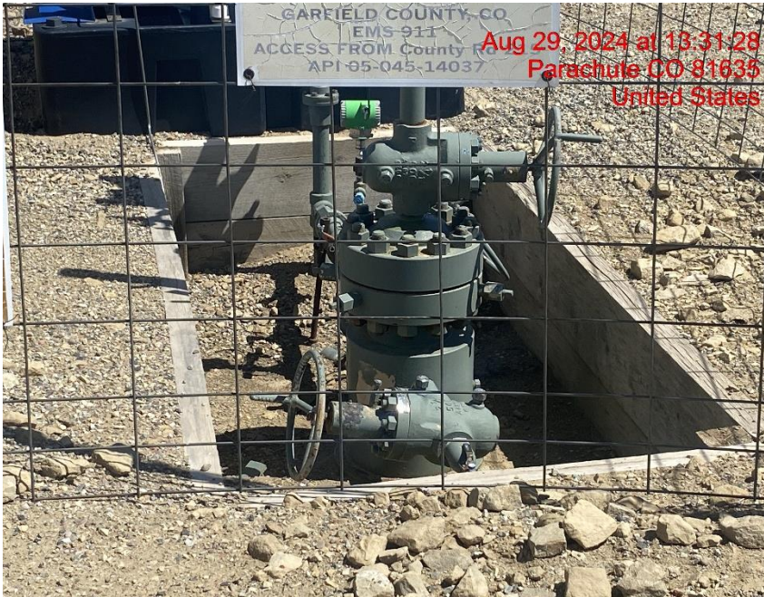
Open Wellhead Cellar – Photo #03174
