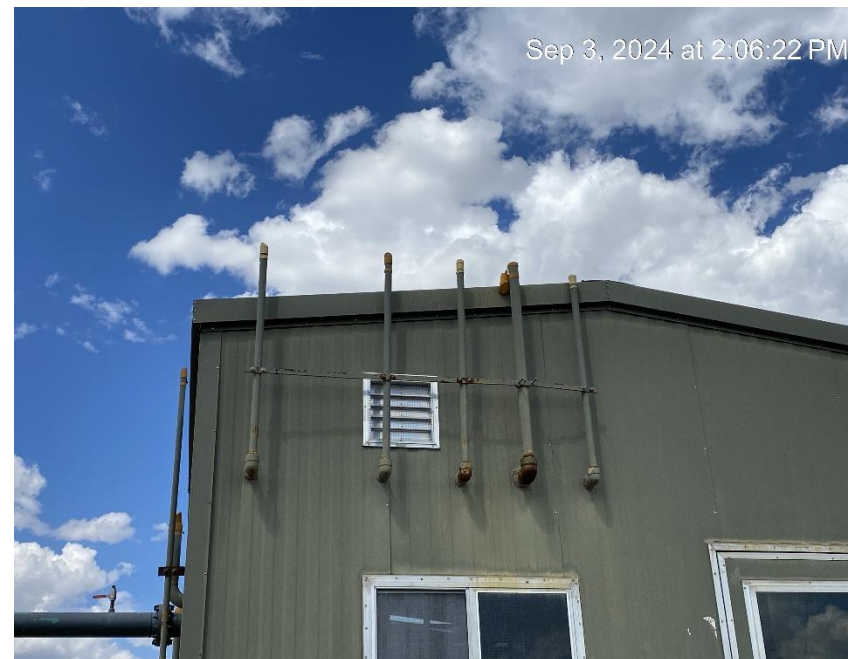
Relief riser missing cap
