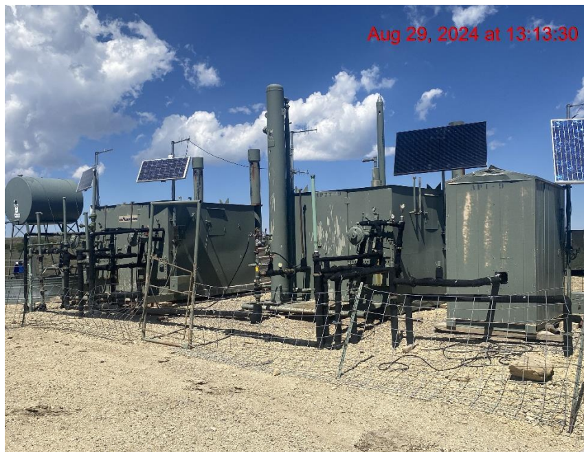
Separators/Gas Meter – Photo #03159
