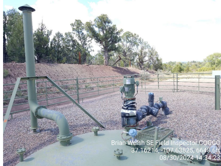
5. Water tank with electric sump pump
