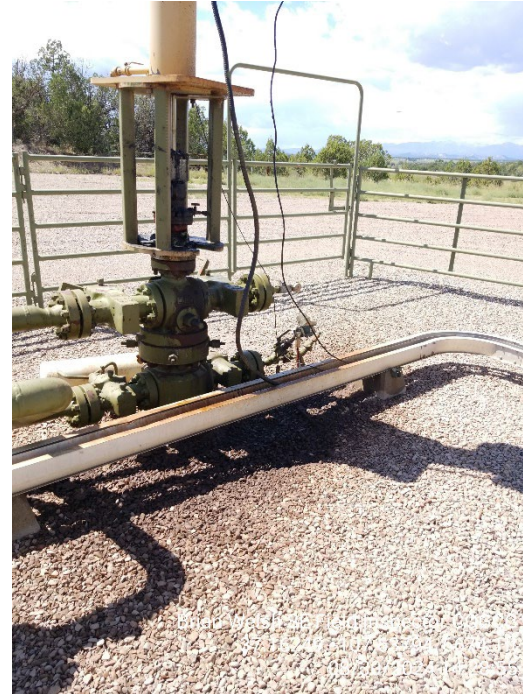
4. Gary Patrick 4 wellhead and pump. Remove and remediate stained rock and soil around wellhead
