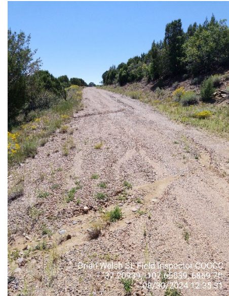
8. Erosion on access near location
