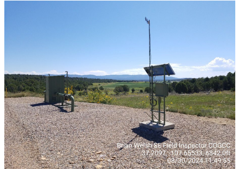
2. Meter shed and telemetry equipment on south side of location is for midstream use
