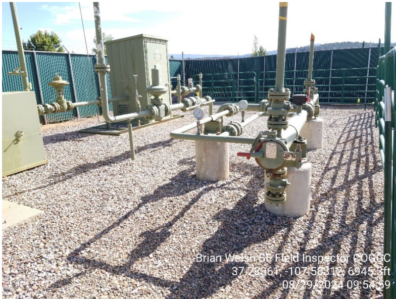
5. Pig station on south side of production equipment
