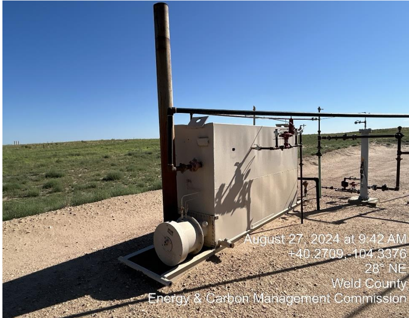
Line Heater. Missing Bird Protector
