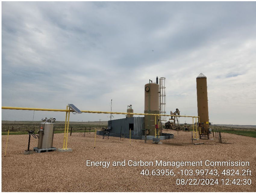
Photo 3 – Heater Treater and ECD
