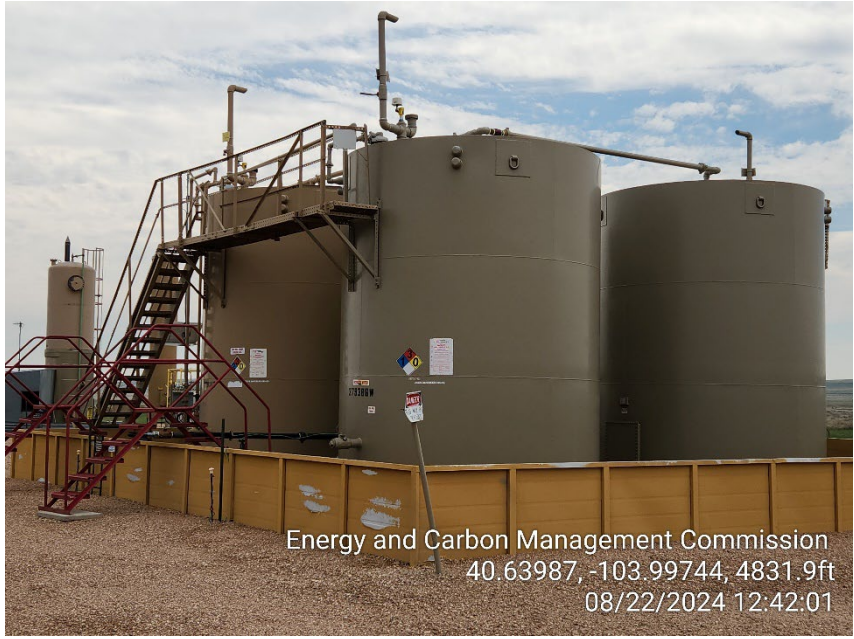
Photo 1 – Tank Battery
