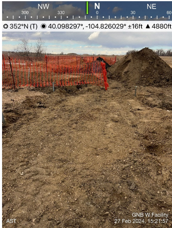
Aboveground Storage Tank Footprint
