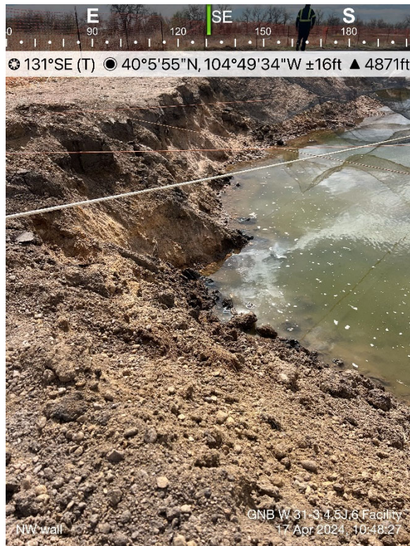
Northwest sidewall of excavation extent
