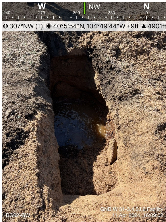
Groundwater at Background Sample BG02
