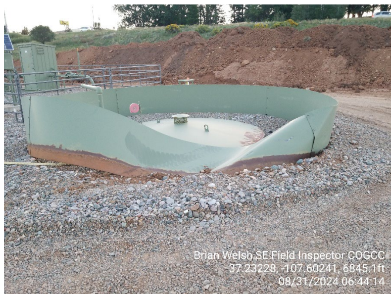
5. Damaged steel ring containment
