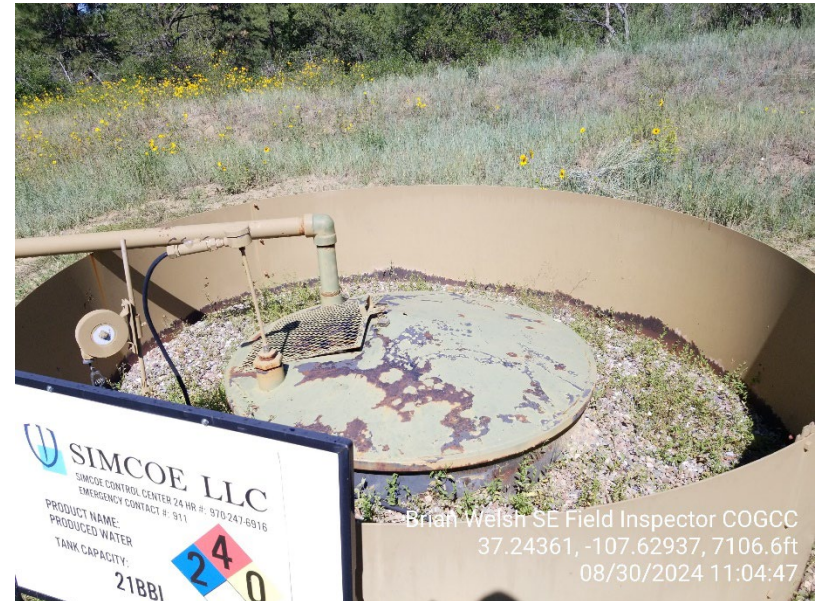
4. Buried water tank
