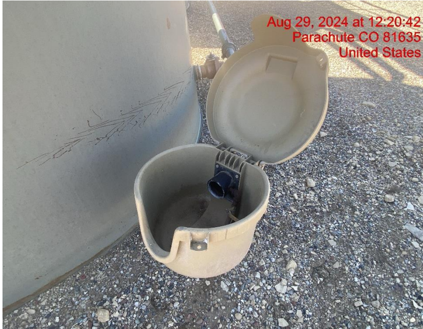
Open-Ended Load Line – Photo #03123
