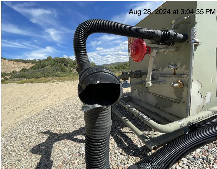
Photo # 7172 Flowline heating insulation open ended/available for entry by wildlife/wildlife hazard
