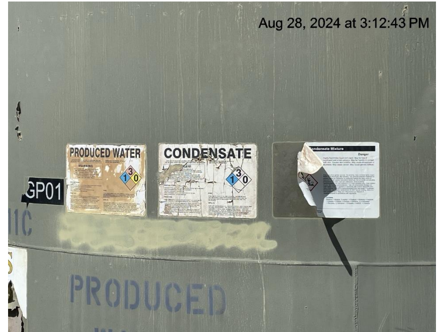
Photo # 7173 Tank labels weathered & 1 label starting to peel
