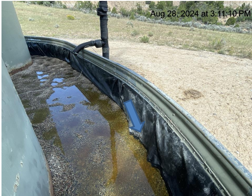
Photo # 7170 Hole in liner/liner needs maintenance
