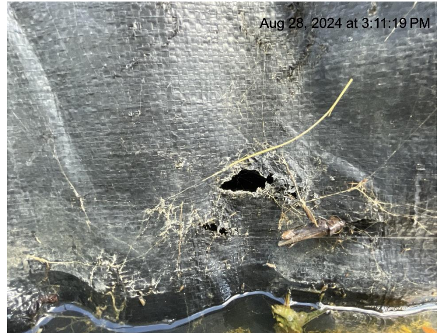
Photo # 7171 Hole in liner/liner needs maintenance
