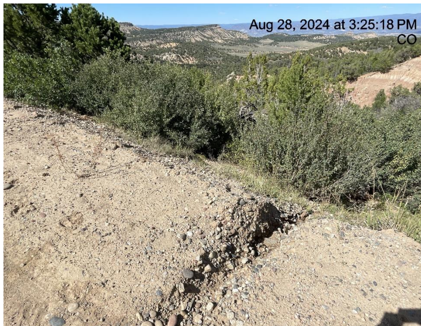
Photo # 7182 Erosion on lease road & transport of sediment off lease road into a vegetated area (approximately 6/10 th of a mile from location)
