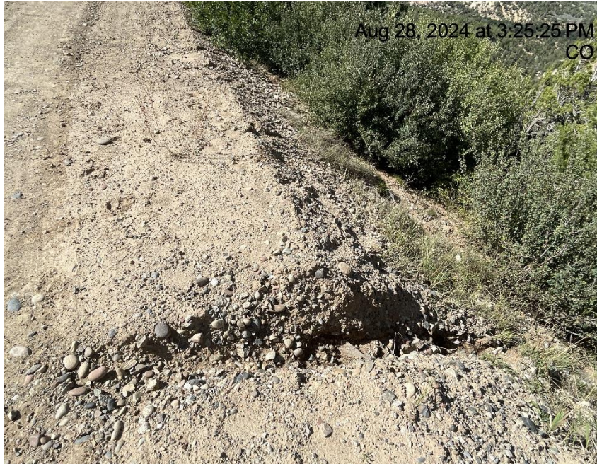
Photo # 7184 Erosion on lease road & transport of sediment off lease road into a vegetated area (approximately 6/10th of a mile from location)
