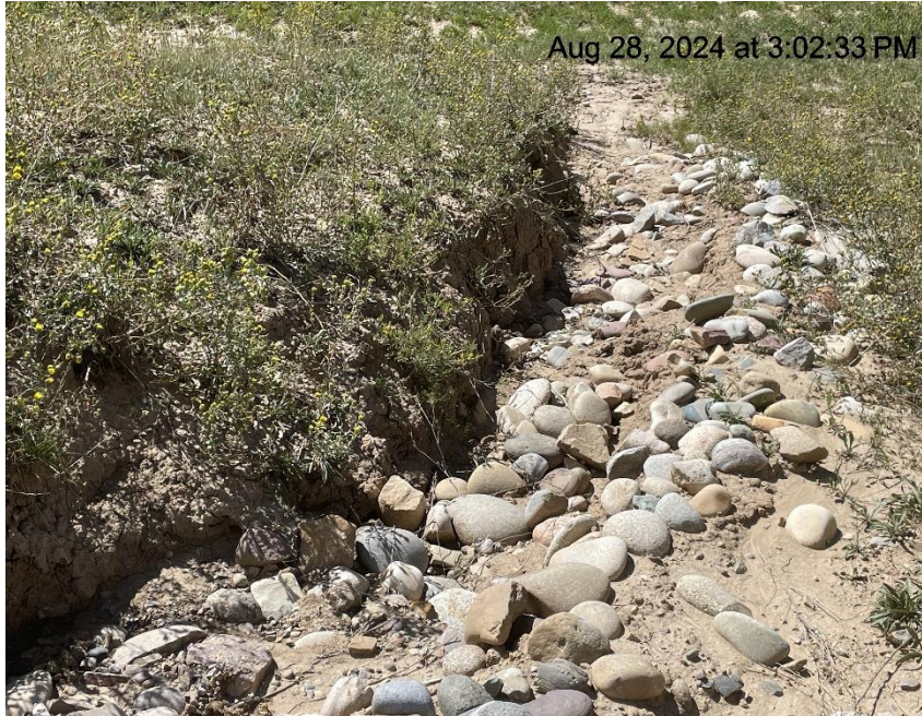
Photo # 7180 Rip Rap Run showing some erosion & sediment buildup (SW corner of location near pig launcher)
