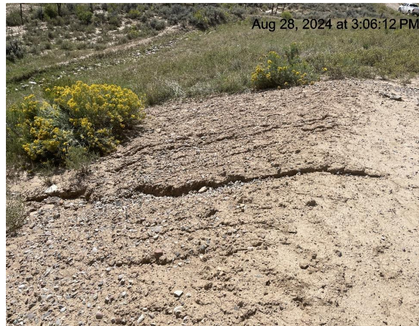
Photo # 7175 Erosion on slope & transport of sediment off location & into a vegetated area (near separator units & Summit Midstream meter house)
