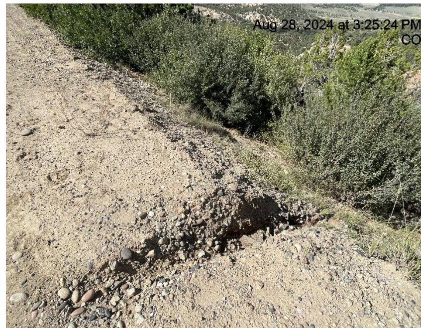
Photo # 7183 Erosion on lease road & transport of sediment off lease road into a vegetated area (approximately 6/10 th of a mile from location)
