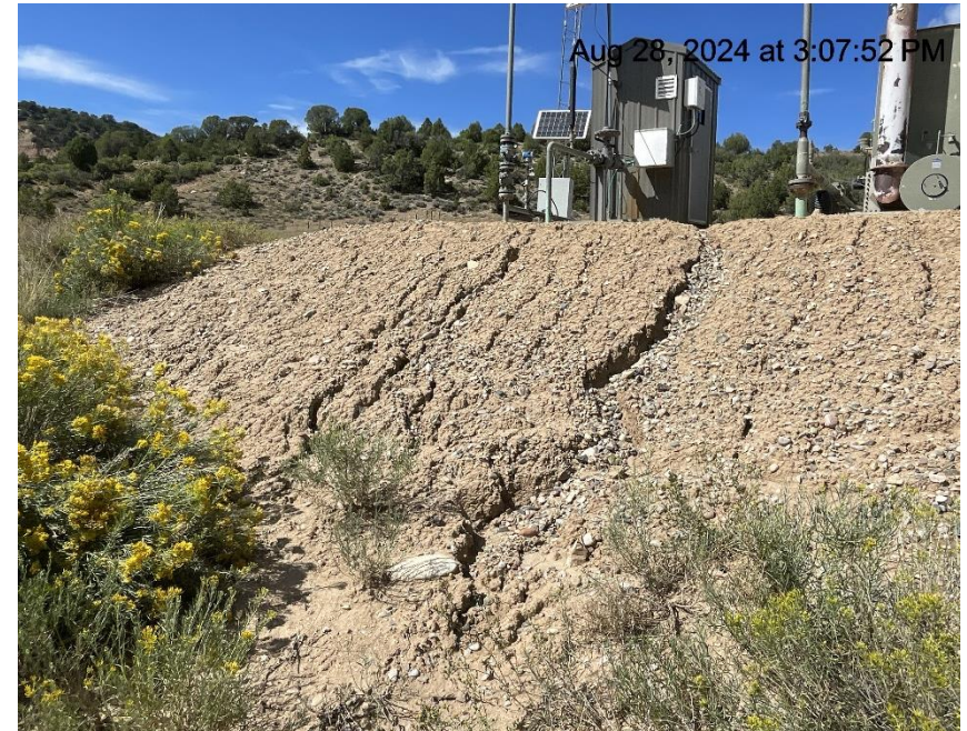
Photo # 7177 Erosion on slope & transport of sediment off location & into a vegetated area (near separator units & Summit Midstream meter house)
