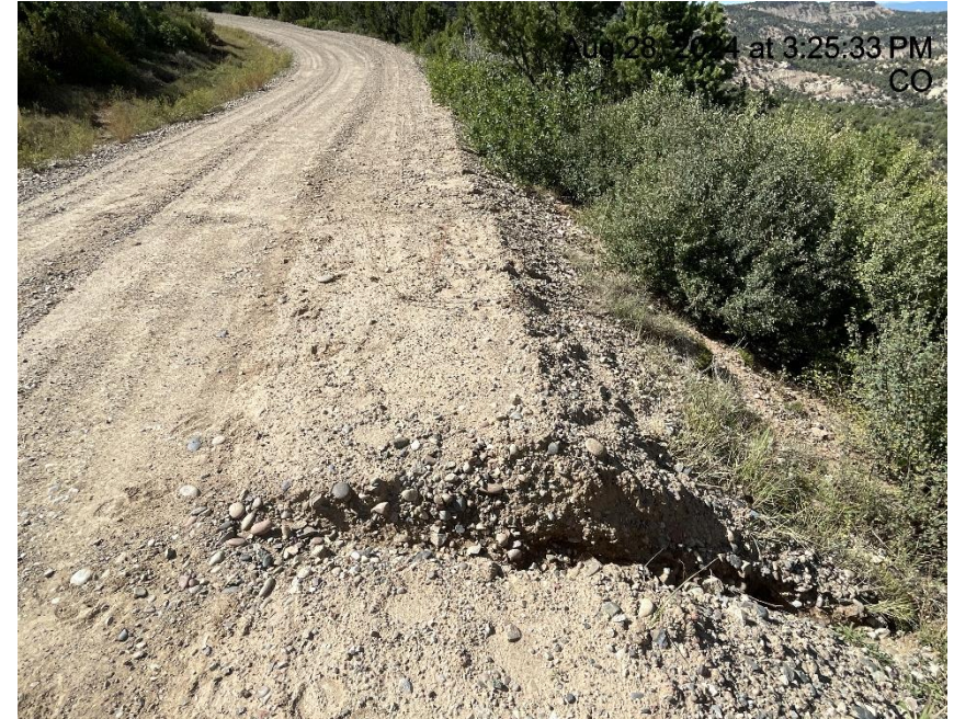
Photo # 7185 Erosion on lease road & transport of sediment off lease road into a vegetated area (approximately 6/10th of a mile from location)
