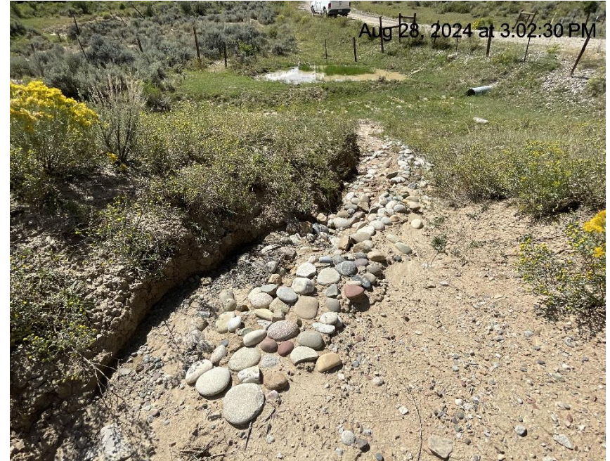
Photo # 7181 Rip Rap Run showing some erosion & sediment buildup (SW corner of location near pig launcher)
