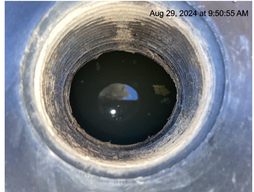
Photo # 7327 Failure to maintain chemical BMP - Chemical tank containment approximately 3/4 full of fluid/BMP insufficient to contain possible spill
