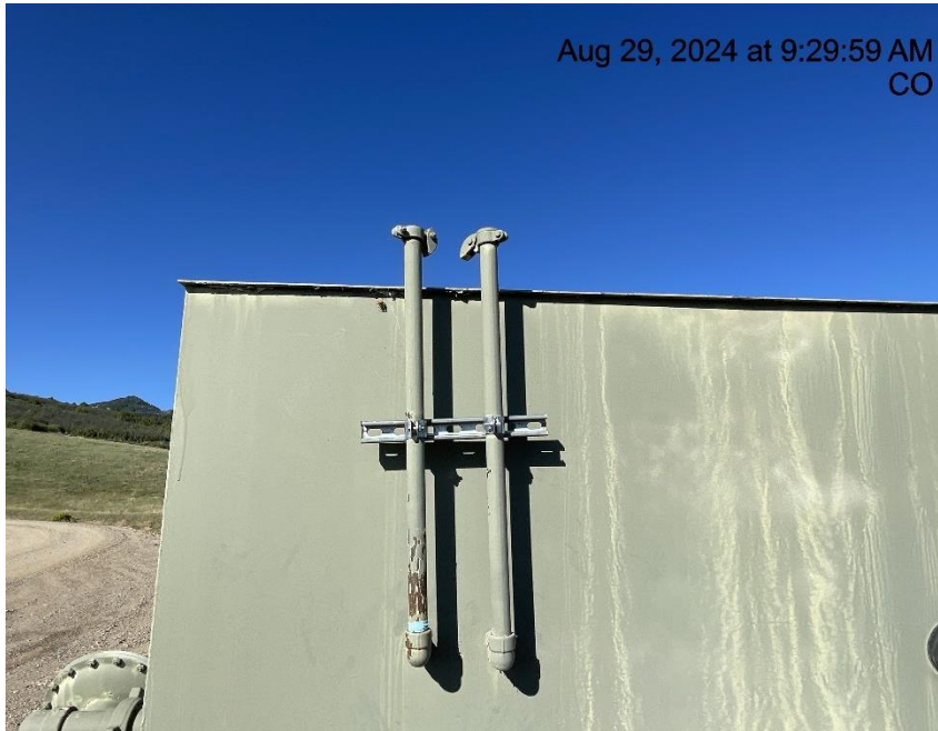
Photo # 7315 PRV vent line does not comply with CECMC pressure safety device rules
