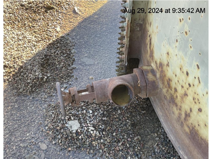
Photo # 7314 Open ended load line
