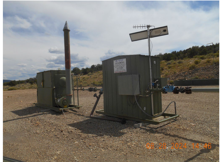
Separator and Meter housing with sign
