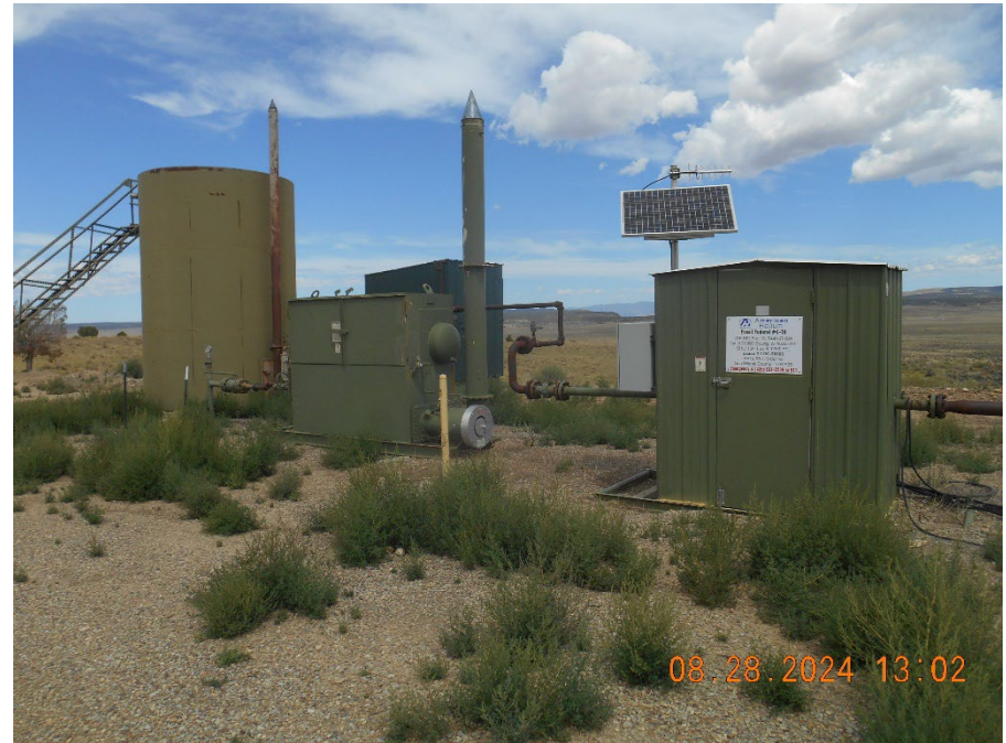
Meter housing, Separator, Fresh water tanks FOSSIL FEDERAL #4-19 API #: 05-113-06118
