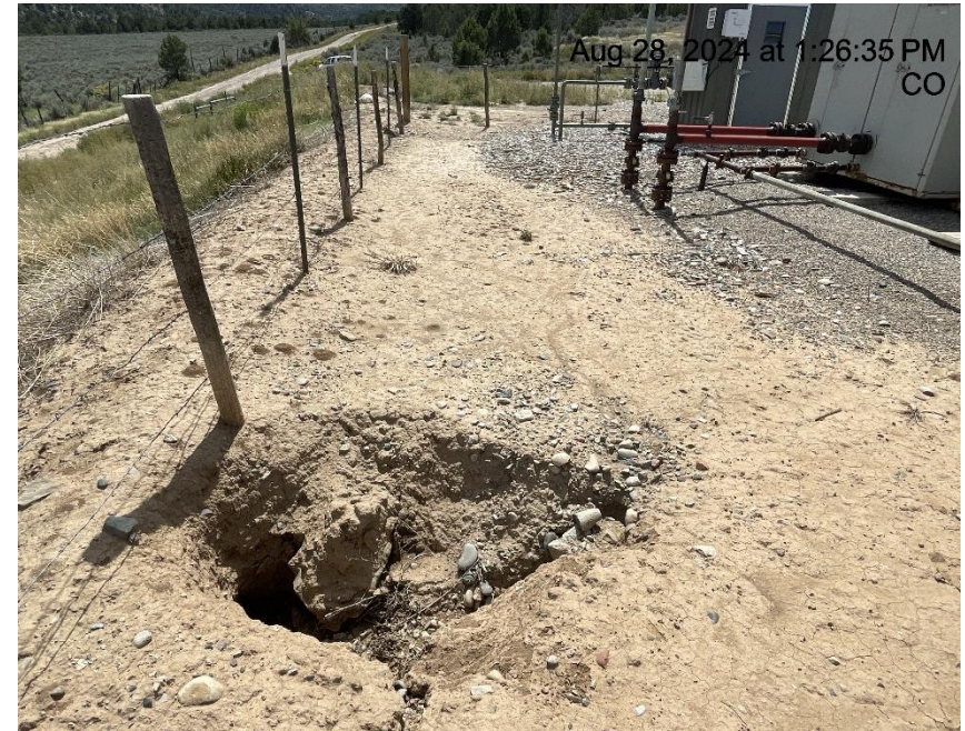
Photo # 6966 Subsidence (area of subsidence is also a safety hazard)
