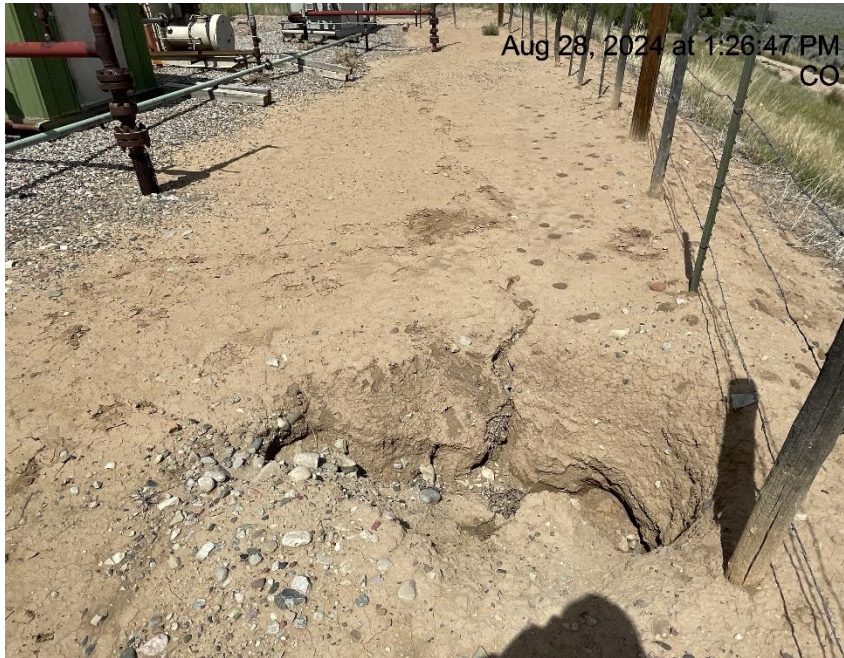
Photo # 6965 Subsidence (area of subsidence is also a safety hazard)
