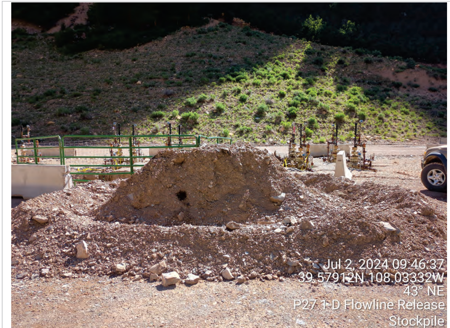
Excavation Stockpile: View Northeast
