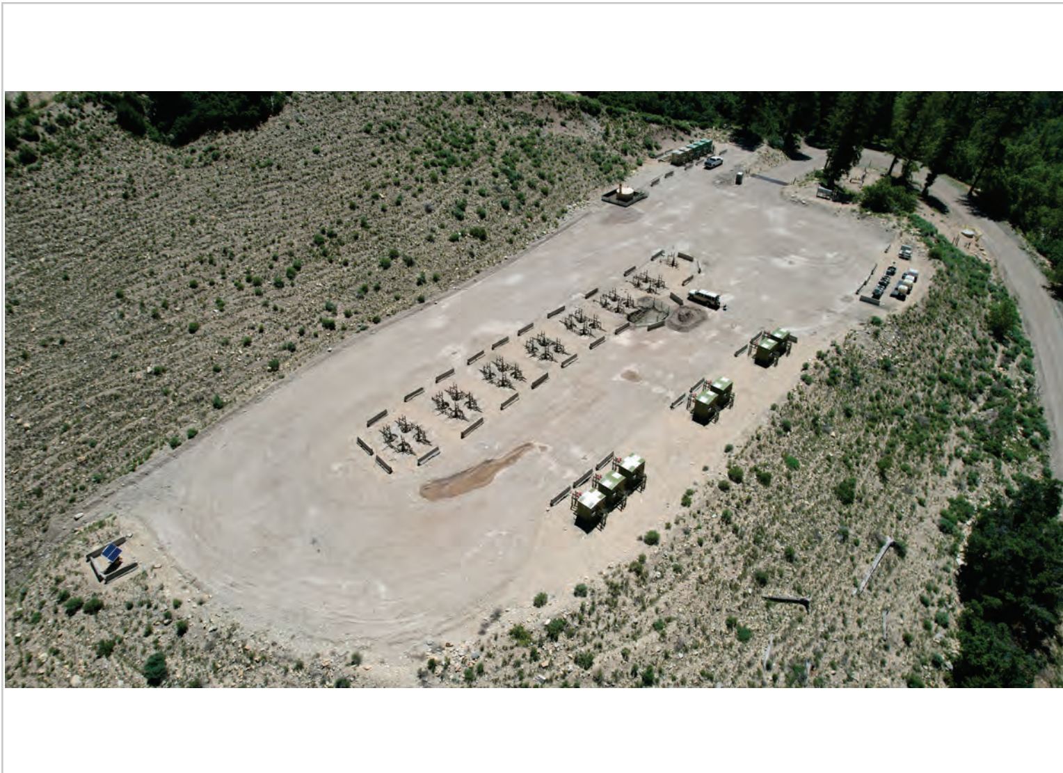
Site Overview: Orientation Southeast
