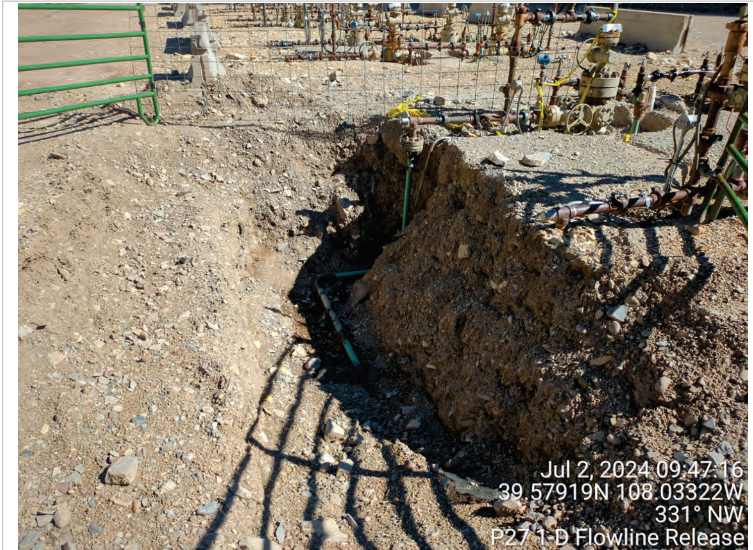
Excavation Overview: View North
