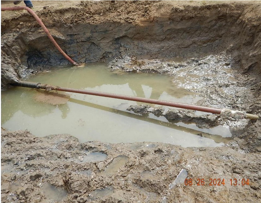
Flowline (off location) repair completed by operator; Approx 20' of 3" fiberglass pipe tied into existing fiberglass flowline (right) and existing 3" carbon steel flowline (left). Flowline enters casing pipe (left).
