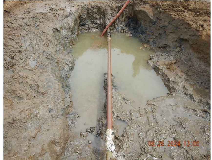
View of flowline pipe repair completed by operator. Looking east.
