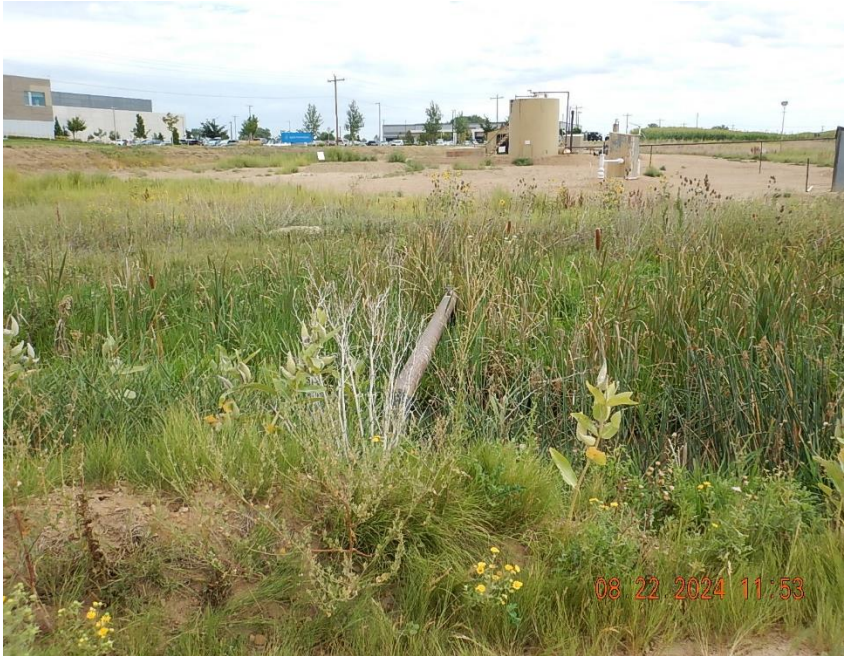
Above ground section of flowline at irrigation ditch crossing. Note: 3" CS flowline is inside 6" CS casing pipe shown.
