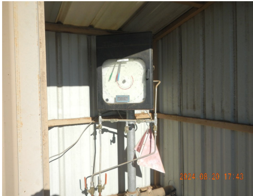
3. Gas meter inside meter shed.
