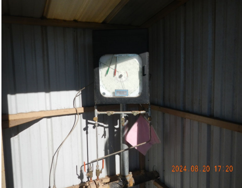
3. Gas meter inside meter shed.
