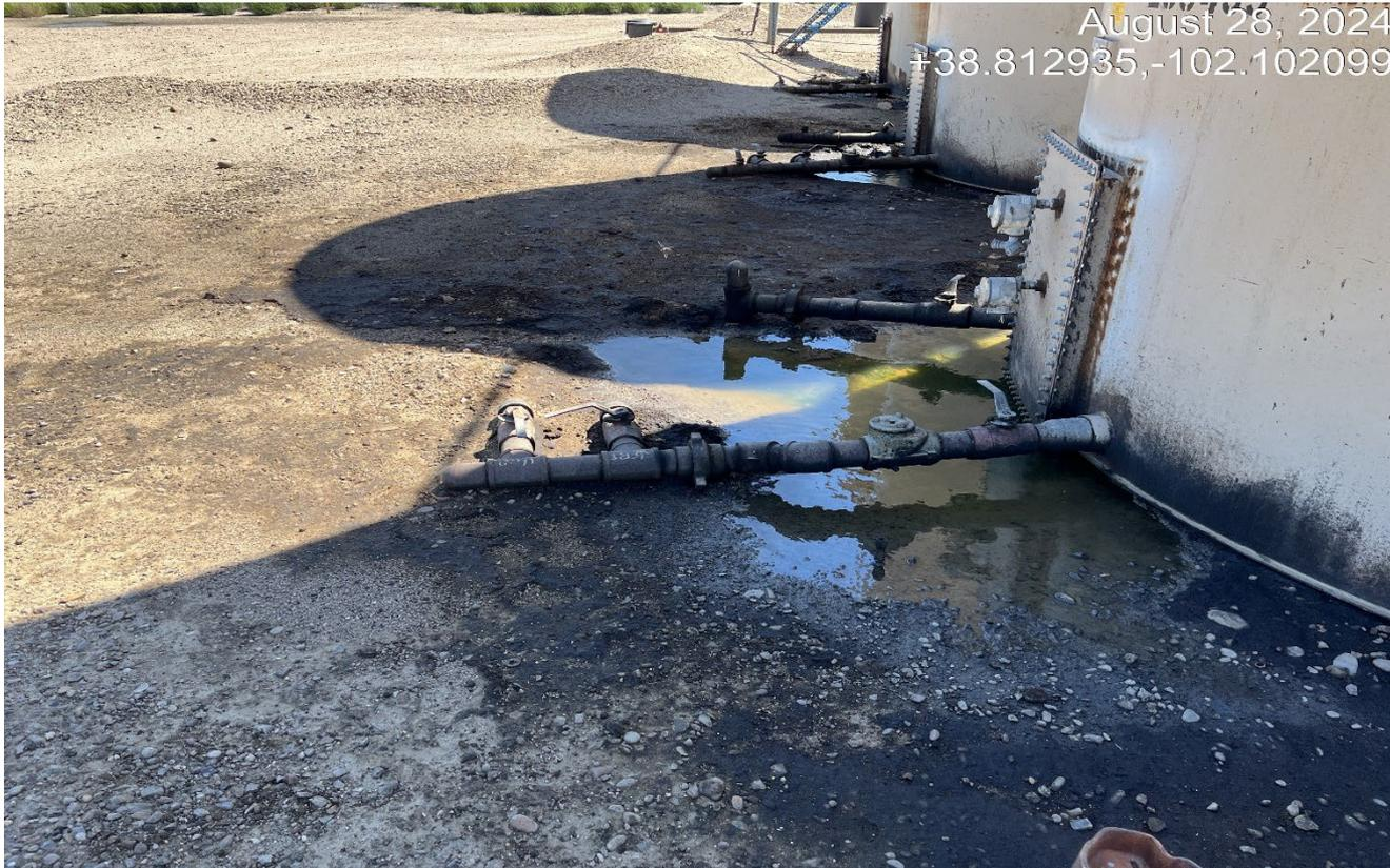
**Photo 5.** Facing east at the north side of the tanks. There is oil saturated soils at the base of the tank that must be cleaned up.
