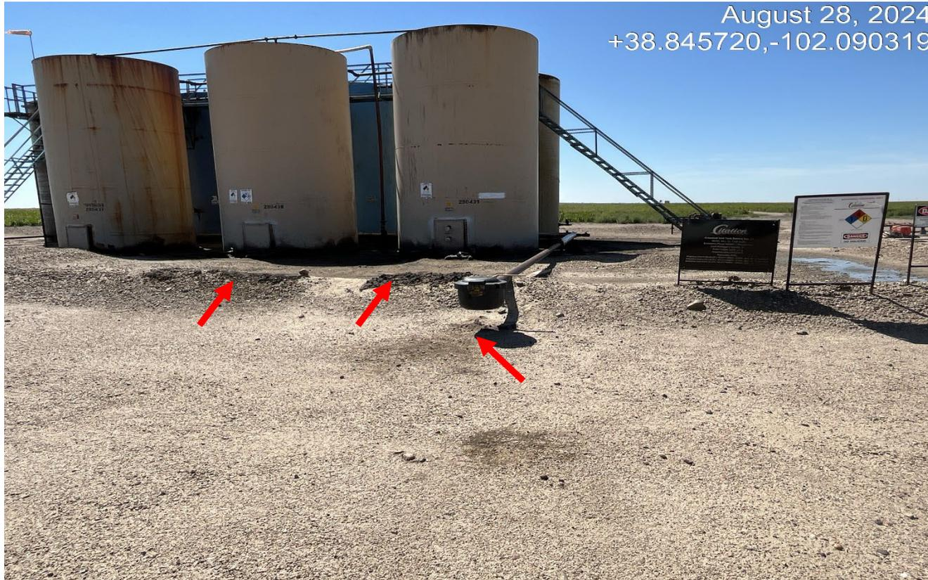
**Photo 1.** Facing southwest toward the Arapahoe Unit Tank Battery/Sec. 27. There is oily material along the berm at red arrows and at the truck load out pipe.
