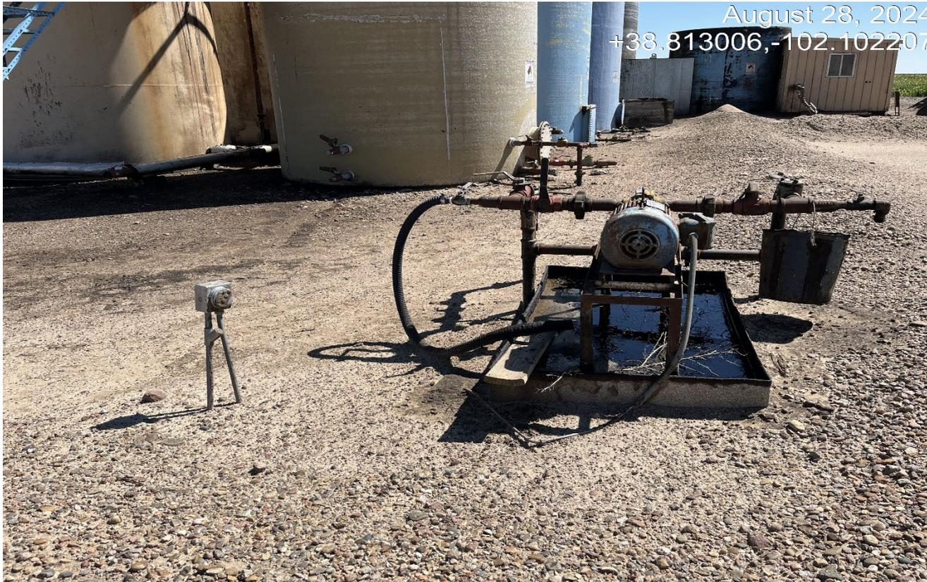
**Photo 2.** This secondary containment is full of oil with no wildlife protections/netting. This needs to be immediately drained and properly disposed.
