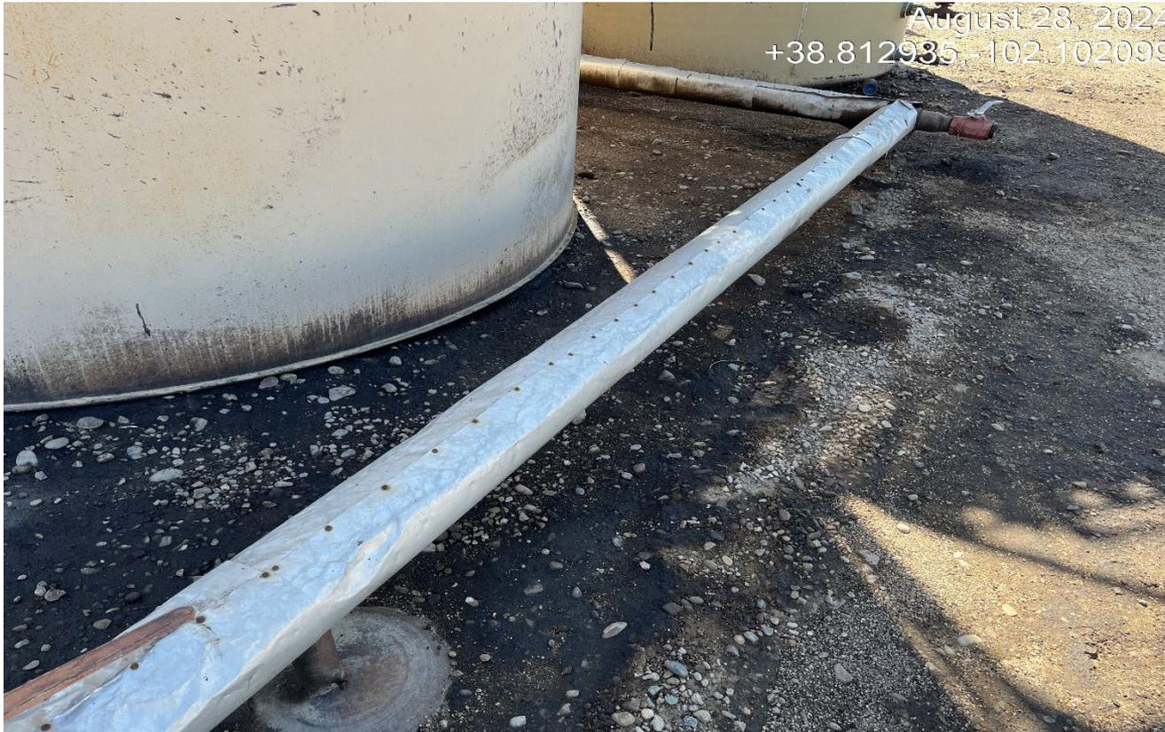
**Photo 4.** There is oil saturated soils at the base of the tank that must be cleaned up.
