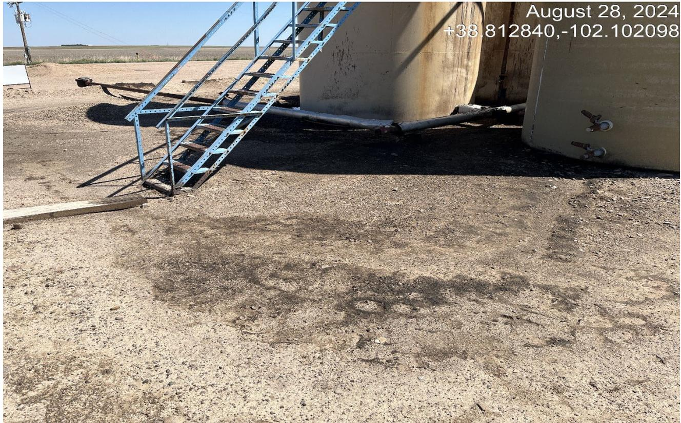
**Photo 3.** On the west side of the tanks there is oil staining from a leak that occurred.
