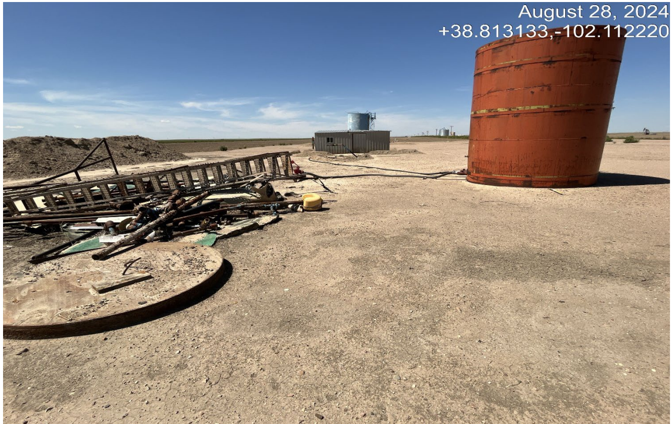
Photo 3. Facing west at the location. The red tank is in use and has no secondary containment or labeling.
