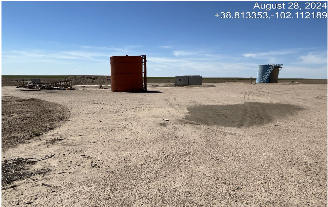
Photo 1. Facing southwest toward the Arapahoe Unit Tank Battery/Sec. 28. There is no secondary containment of the red tank.
