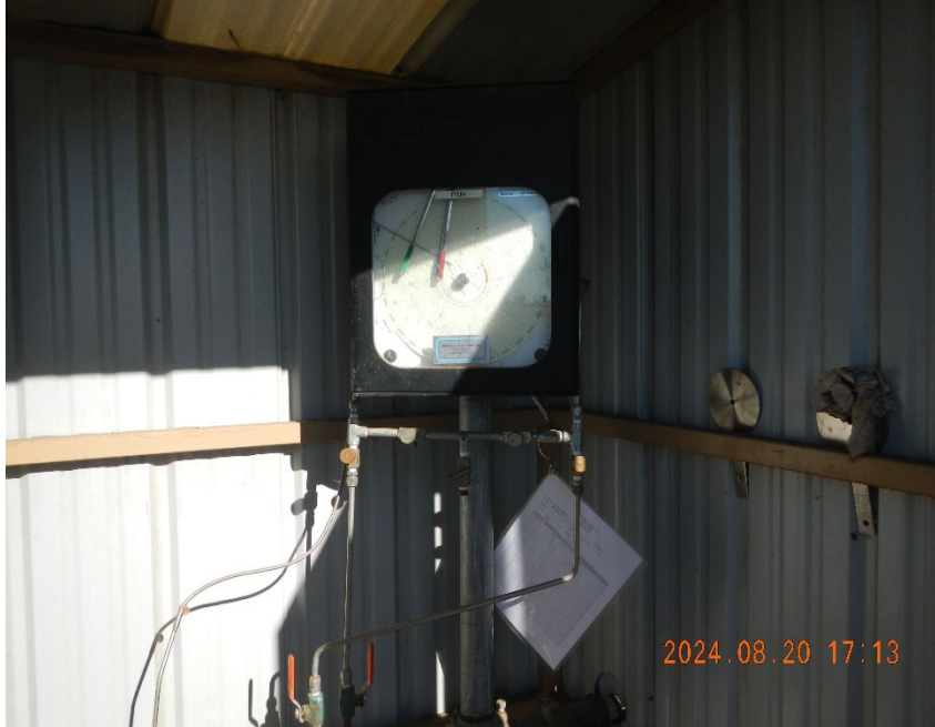
3. Gas meter inside meter shed.
