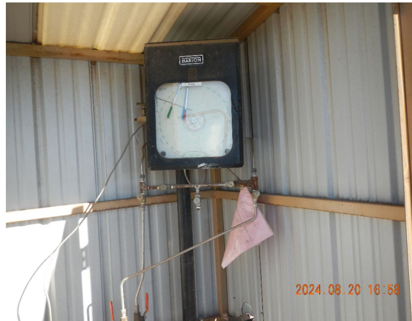
4. Gas meter inside meter shed.
