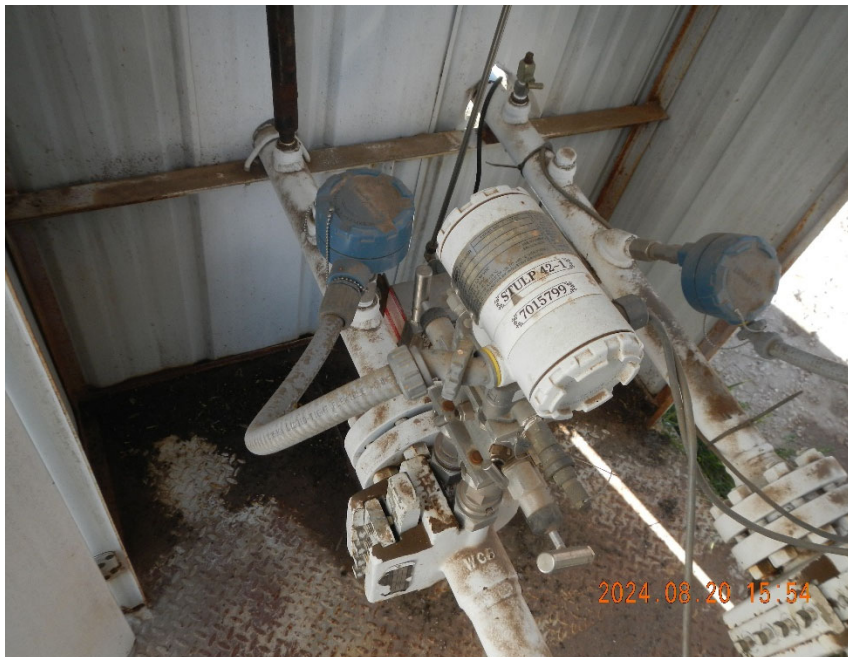
5. Gas meter inside remote meter shed.
