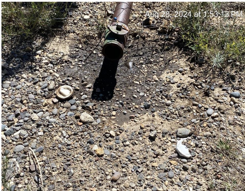
Debris. Stained soil. Open end load line.
