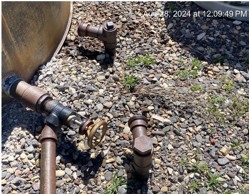
Lines open to wildlife. Staining.
