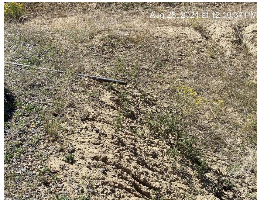
Drain line open to wildlife
