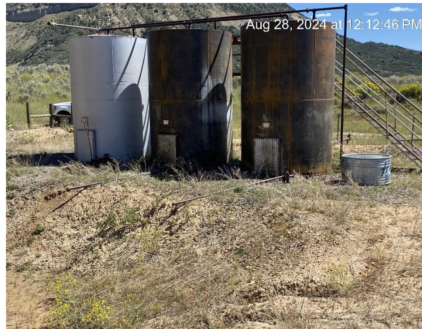
Tank battery with open drains to pit
