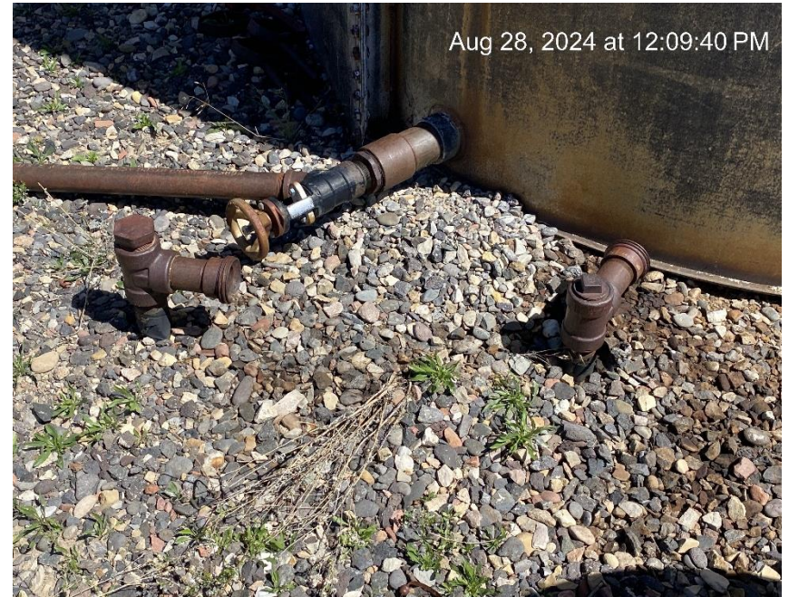
Lines open to wildlife. Staining.
