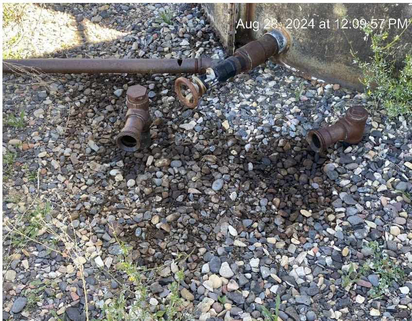
Lines open to wildlife. Staining.
