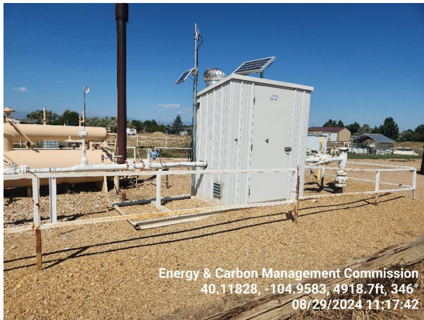
Photo7 Gas Meter Run SI, LOTO card indicates current calibration
