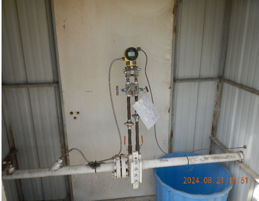
5. Gas meter inside meter shed.
