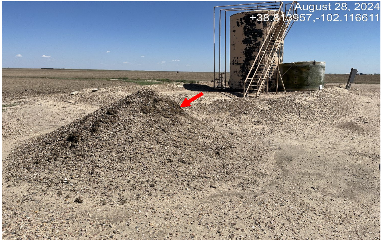
Photo 3. Facing northeast at the tank battery at the north side of the location. There is a pile of impacted material stored on location outside of secondary containment that must be removed and properly disposed.
