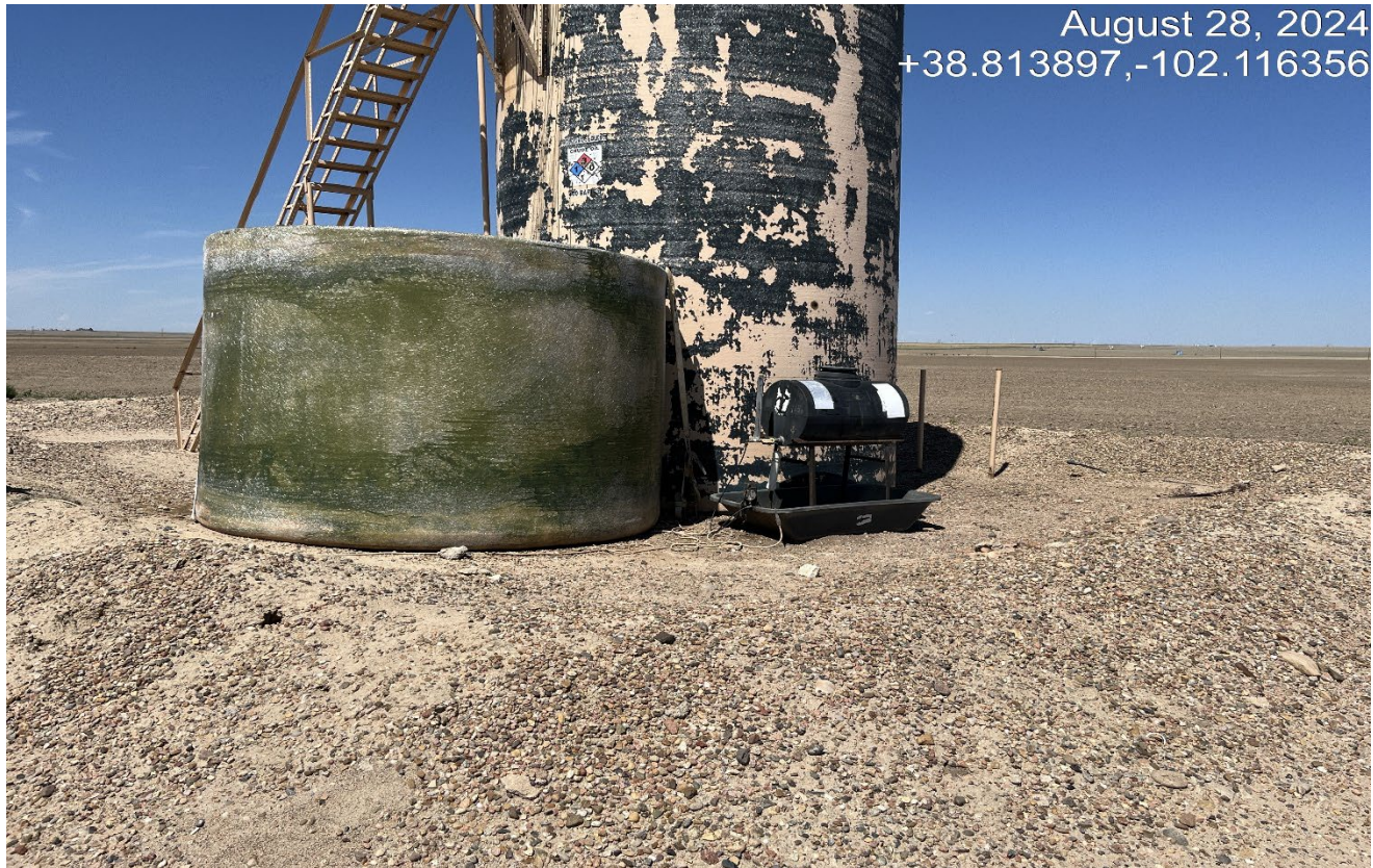
Photo 4. The tank labeling is faded and/or missing.
