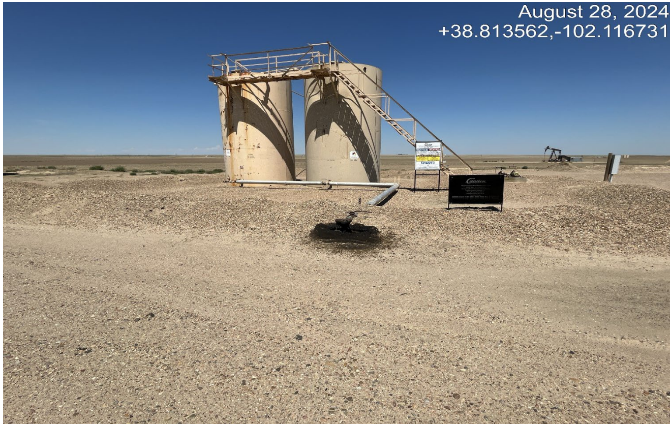
Photo 1. Facing northwest toward the Arapahoe Unit Tank Battery. There is an oil leak out at the discharge pipe that must be controlled and cleaned up.
