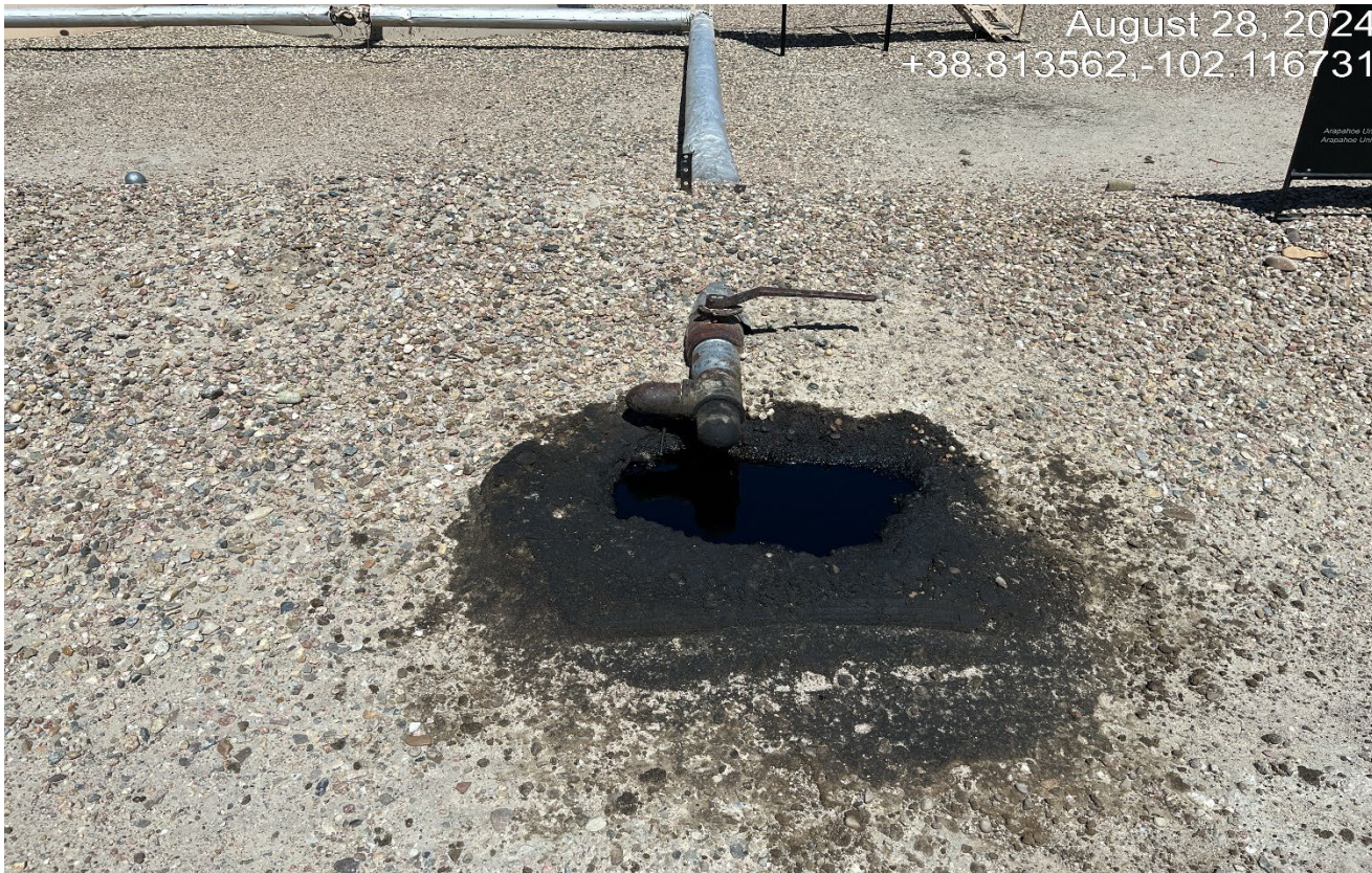
Photo 2. There is a puddle of oil at the discharge pipe that must be controlled, cleaned up, and contained.
