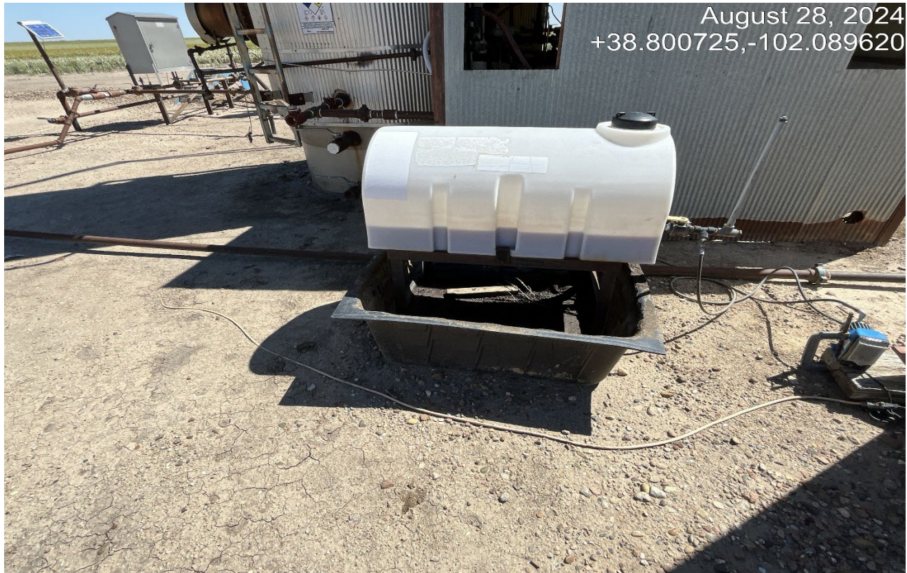
Photo 8. This chemical containment has oily sludge and no wildlife protections. The labels are faded and need to be updated.
