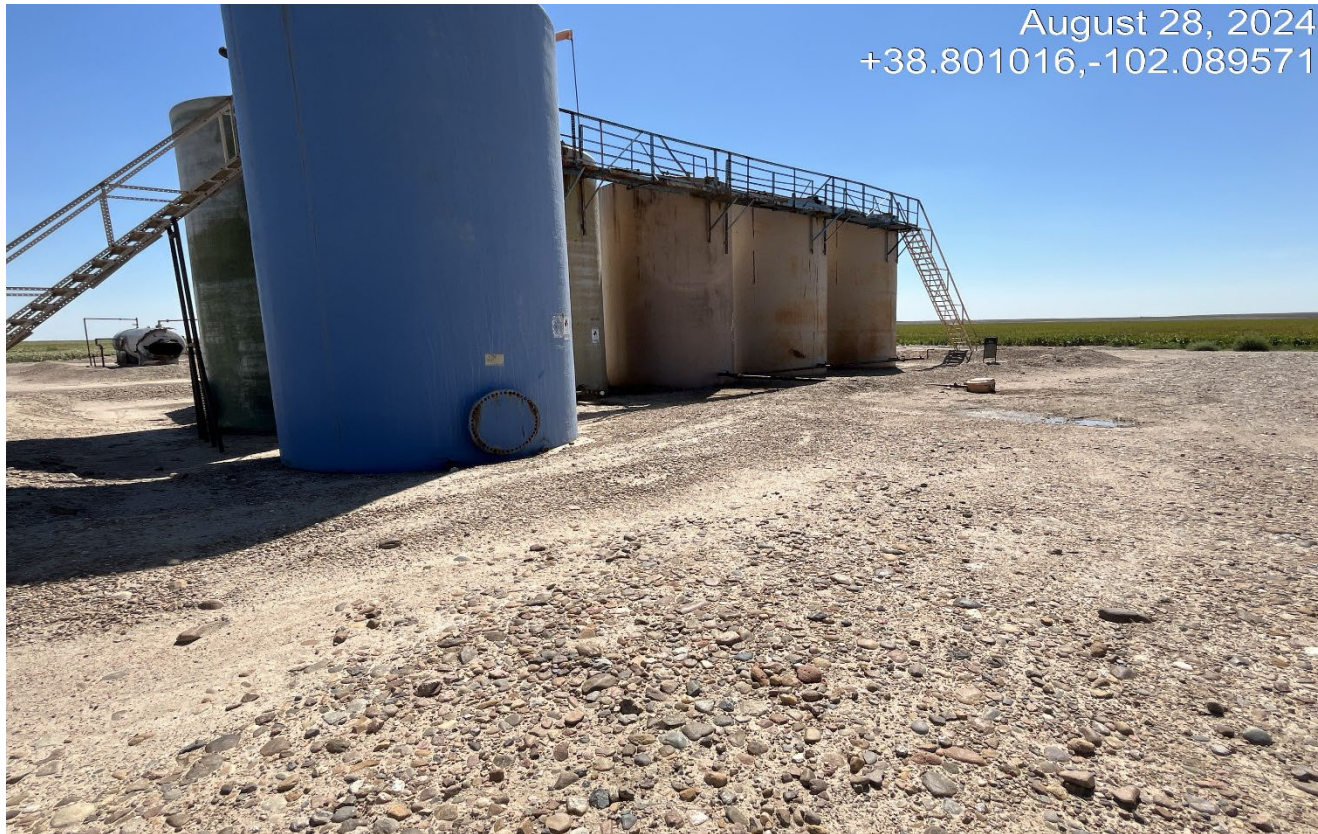
Photo 1. Facing southeast toward the Arapahoe Unit Tank Battery. Some of the tanks have missing or faded labeling.
