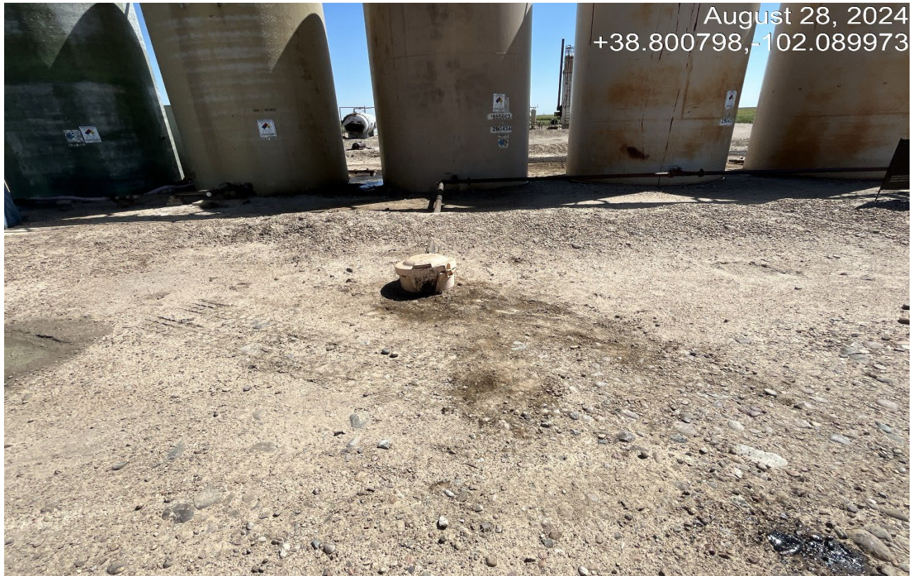
Photo 2. There are some oil stained soils at the pipe outlet that need to be cleaned up.
