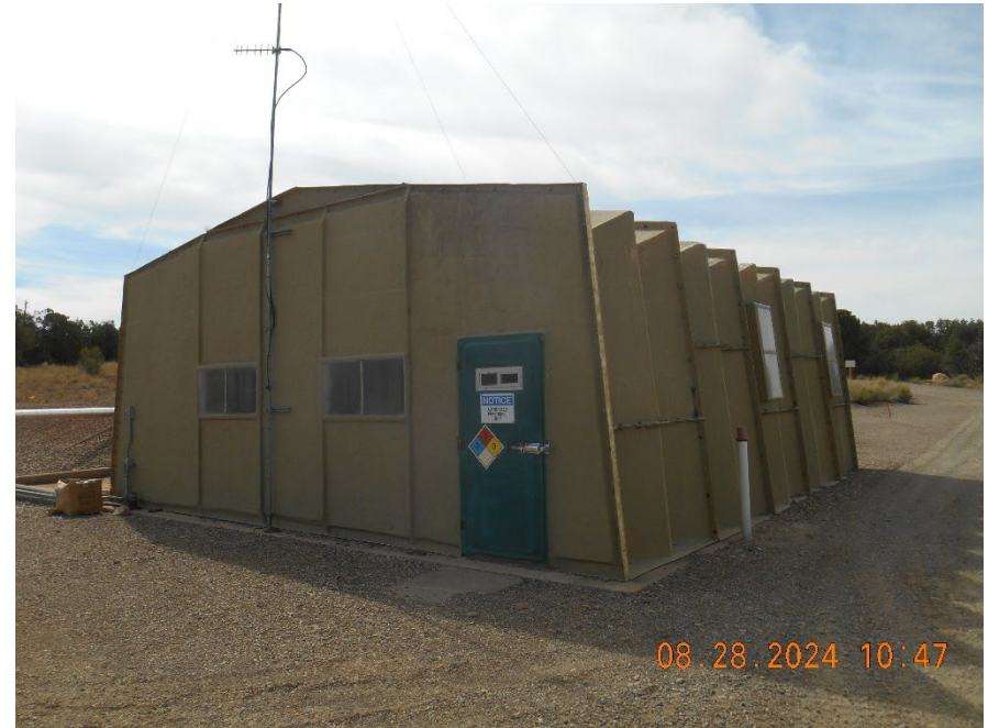
Manifold Housing and control station
