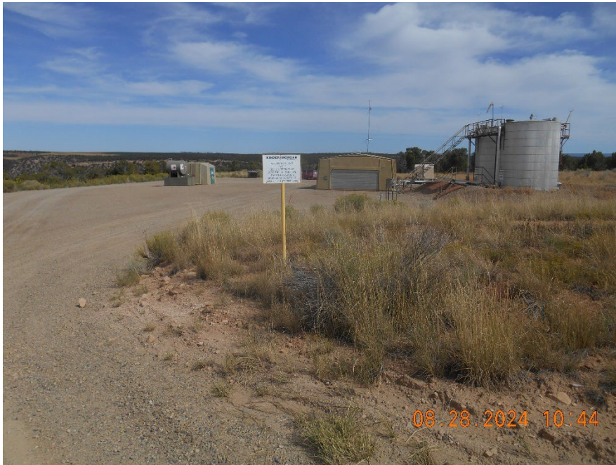
Location overview looking N
