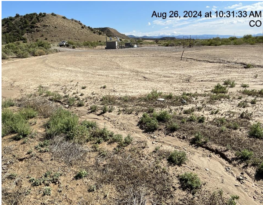
Photo # 6453 Erosion & transport of sediment off location & into a vegetated area/failure to minimize erosion & transport of sediment
