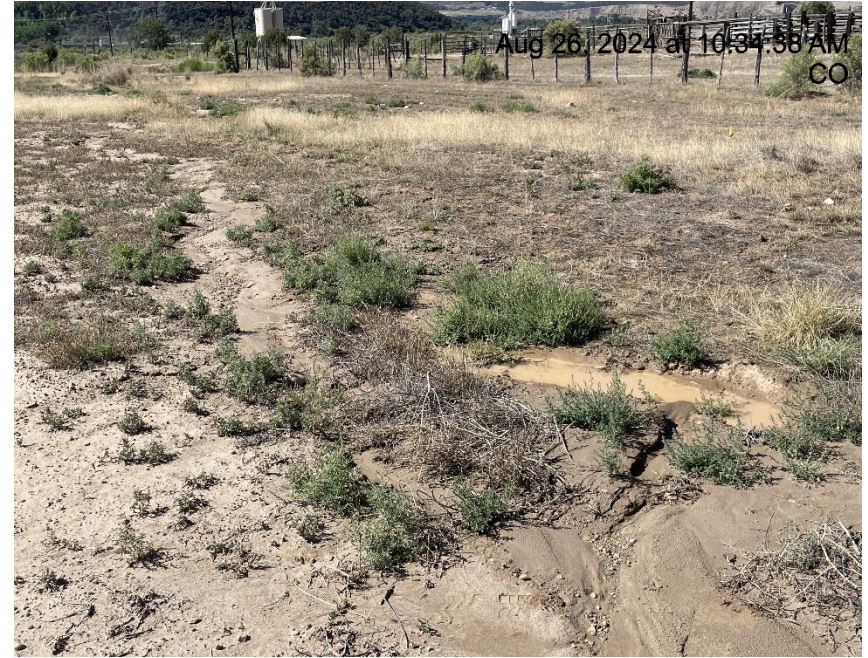
Photo # 6458 Erosion & transport of sediment off location & into a vegetated area/failure to minimize erosion & transport of sediment
