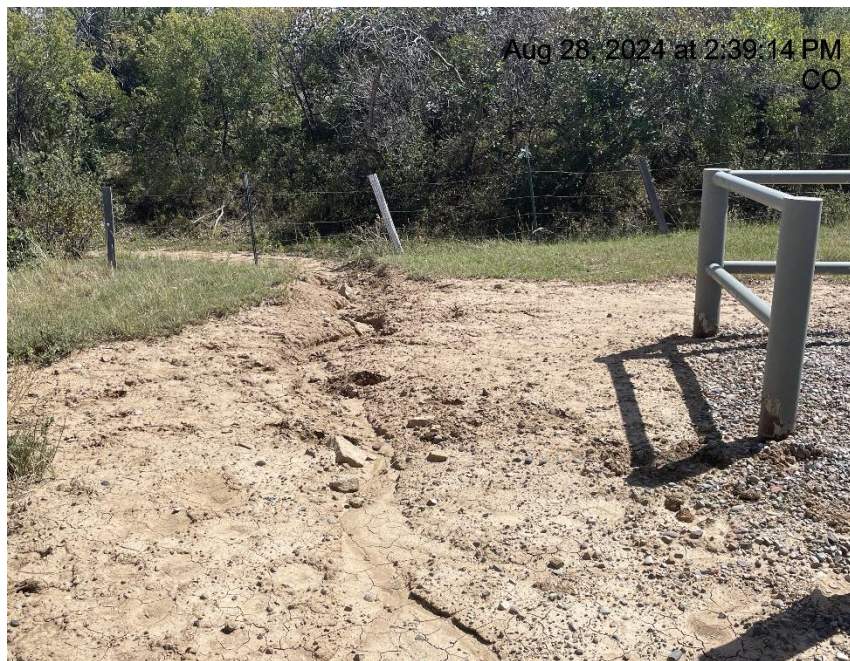
Photo # 7118 Erosion & transport of sediment off location/failure to minimize erosion & transport of sediment (near pig station at entrance to location)
