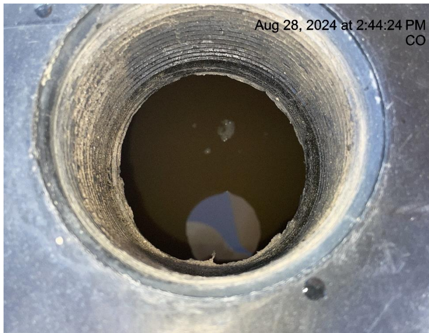
Photo # 7116 Failure to maintain chemical BMP - Chemical tank containment approximately 3/4 full of fluid/BMP insufficient to contain possible spill.
