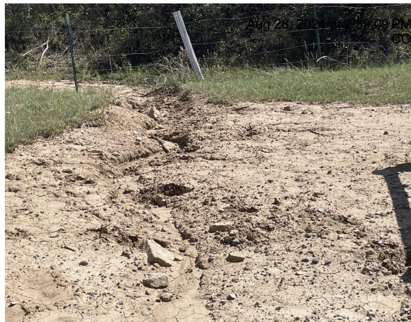
Photo # 7119 Erosion & transport of sediment off location/failure to minimize erosion & transport of sediment (near pig station at entrance to location)
