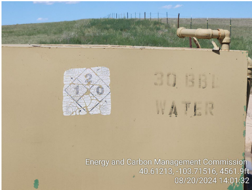
Photo 5 – Labels fading – Replace soon
