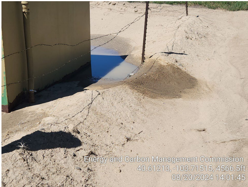
Photo 7 – Water Tank – Berms Inadequate
