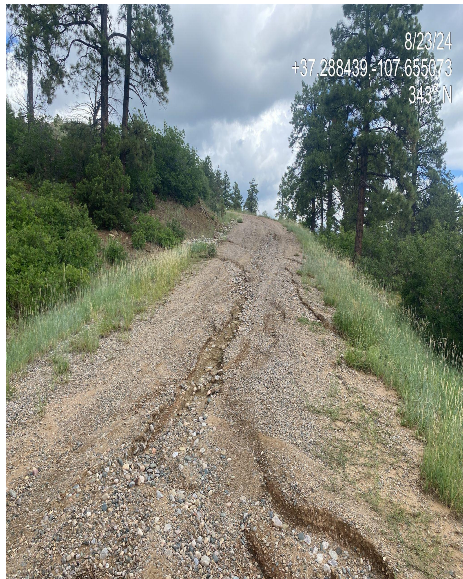
Photo 3. View of rutting/erosional channels along the access road. Additional stabilization, storm water BMP maintenance is needed to minimize degradation to access road.
