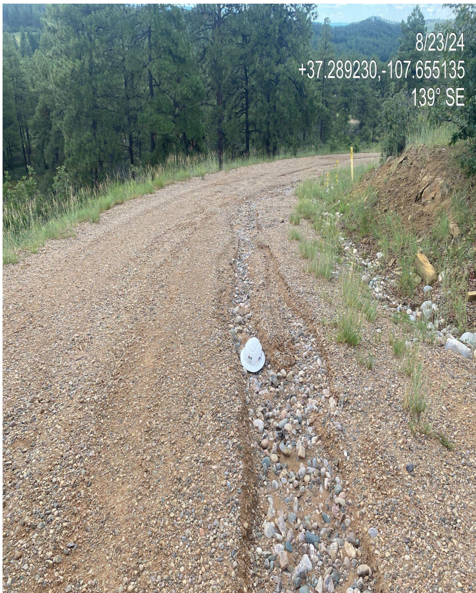
Photo 3. View of rutting/erosional channels along the access road. Additional stabilization, storm water BMP maintenance is needed to minimize degradation to access road.
