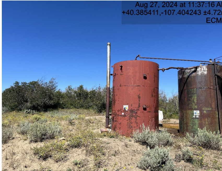
Unknown if bird protection is in place on tank heater vent
