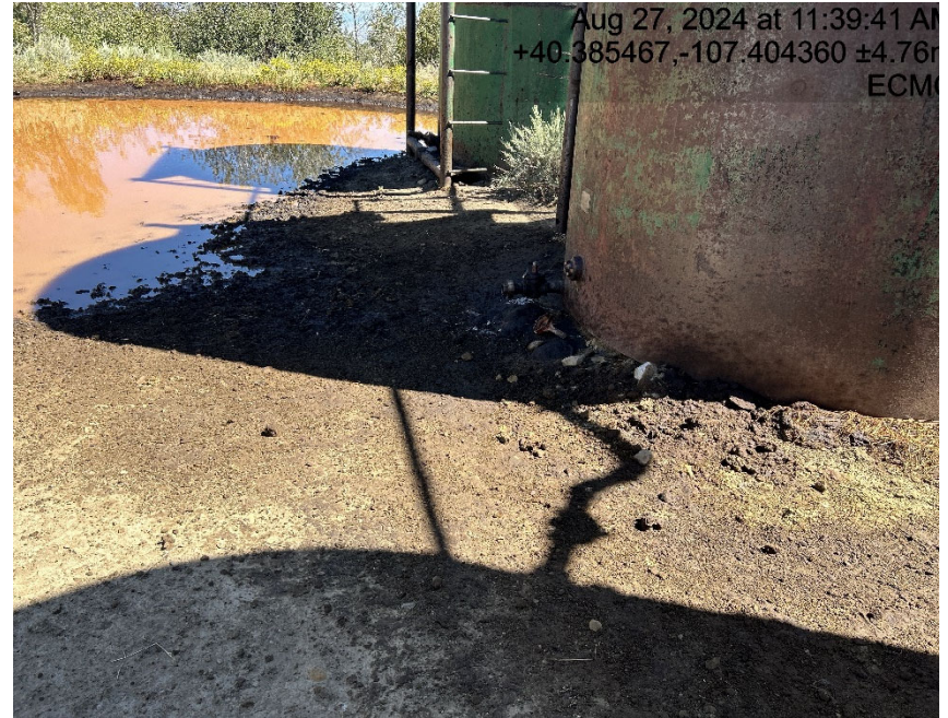
Oil and stained materials in secondary containment.
