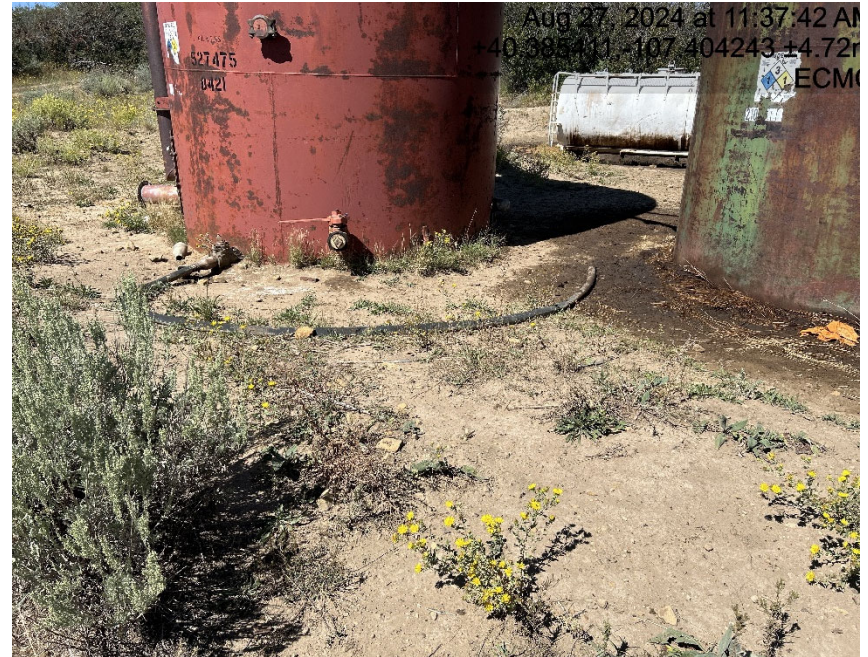
Oil and stained materials in secondary containment. Open ended hose connected to tank
