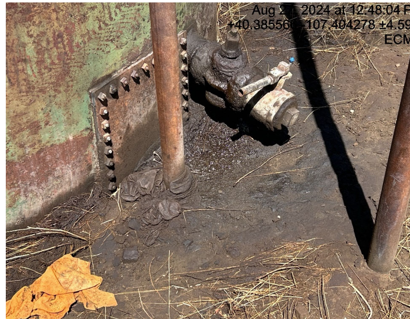
Oil and stained materials in secondary containment.
