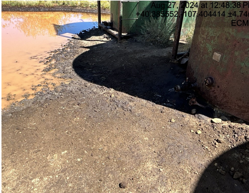
Oil and stained materials in secondary containment.
