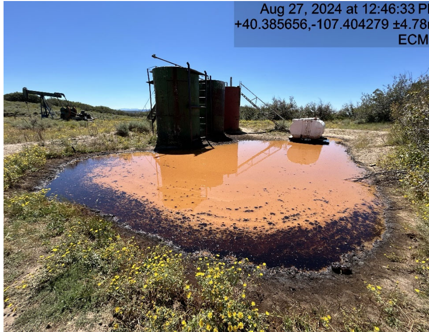
Oil and stained materials in secondary containment
