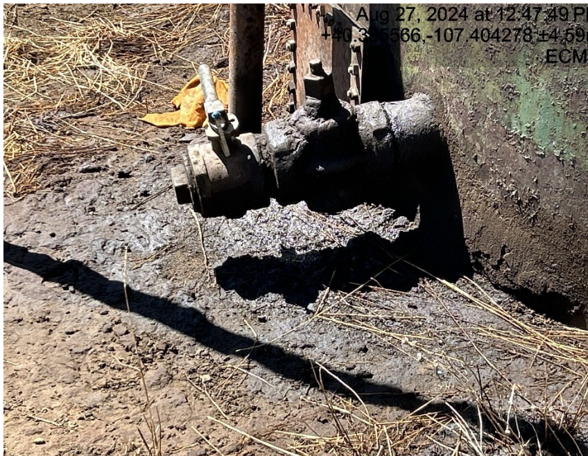
Oil and stained materials in secondary containment.
