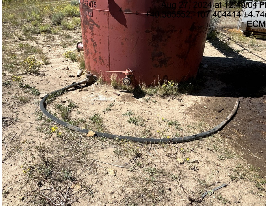
Oil and stained materials in secondary containment. Open ended hose connected to tank
