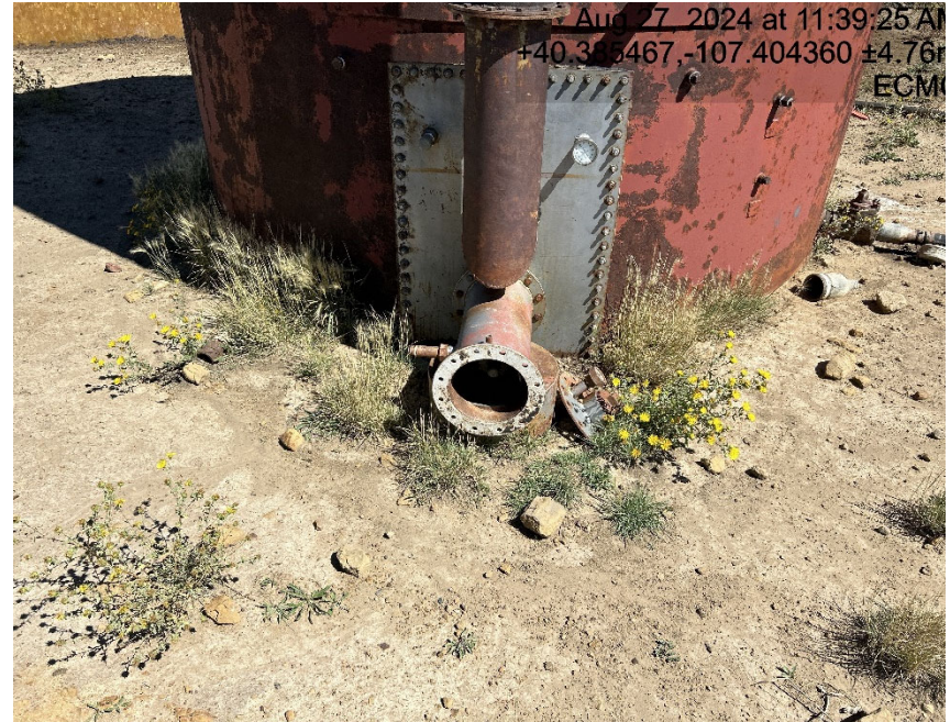
Tank heater is disconnected but open for wildlife to enter
