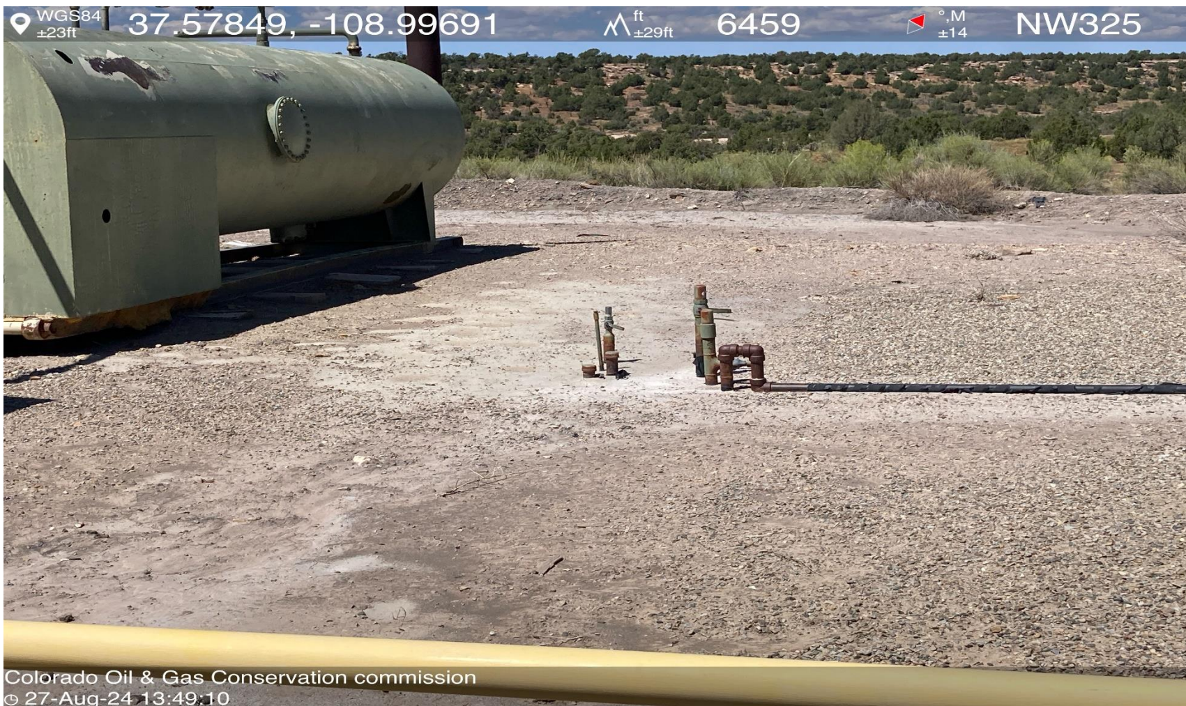
PHOTO 12: UNUSED EQUIPMENT (5 2" AND 1 1" RISERS NEAR HEATED SEPARATOR). REMOVE OR MARK RISERS FOR WHAT THEY CARRY (IE. WATER, GAS ECT.). PER RULE 606.
