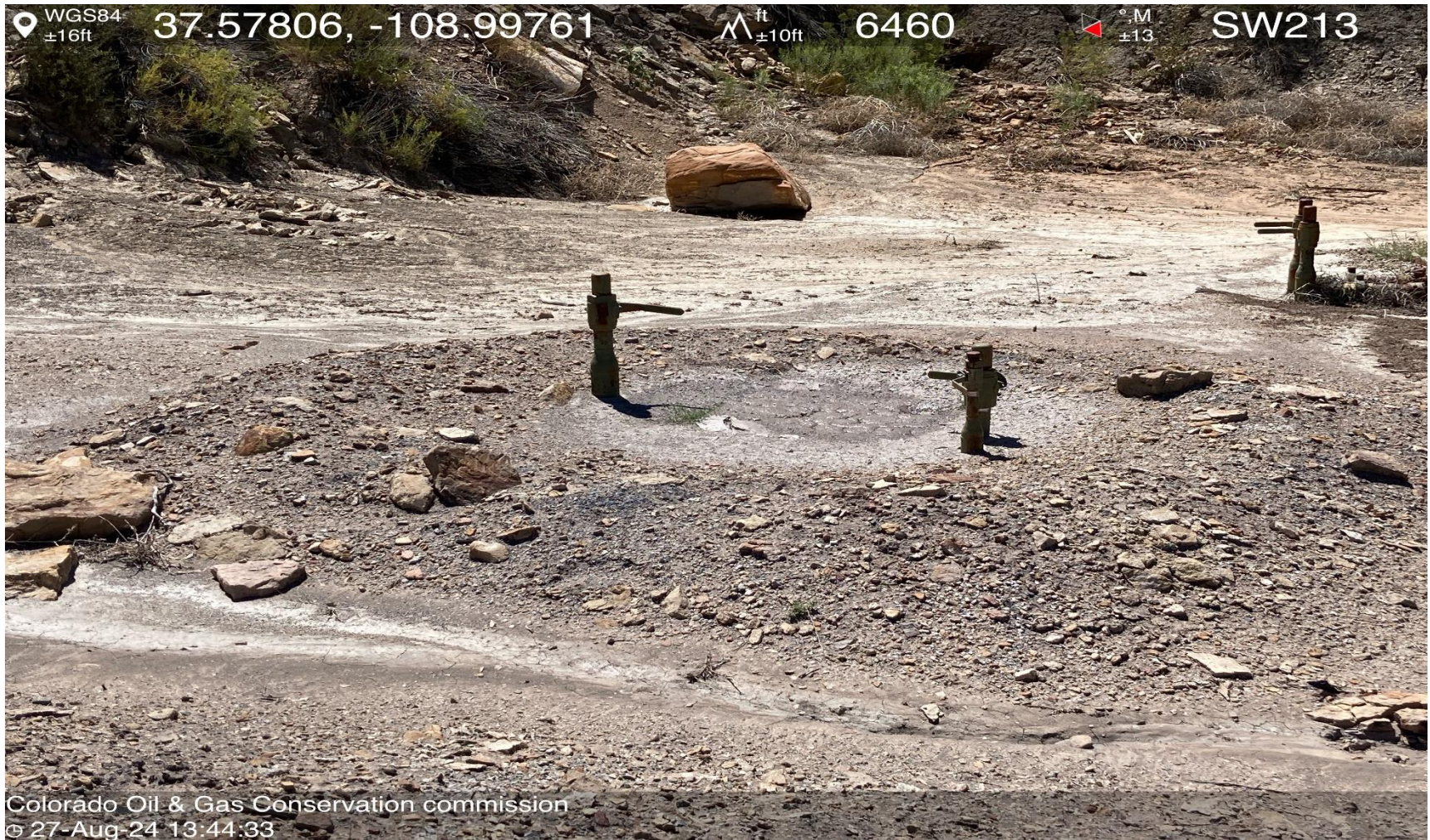
PHOTO 9: UNUSED EQUIPMENT (2 2" RISERS AND 1 1 ¾" RISER NEAR CRUDE OIL TANKS). REMOVE OR MARK RISERS FOR WHAT THEY CARRY (IE. WATER, GAS ECT.). PER RULE 606.
