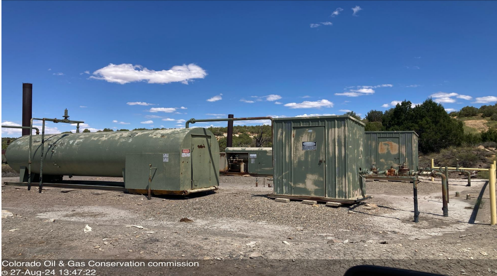
PHOTO 7: HEATED SEPARATORS AND METER HOUSES.
