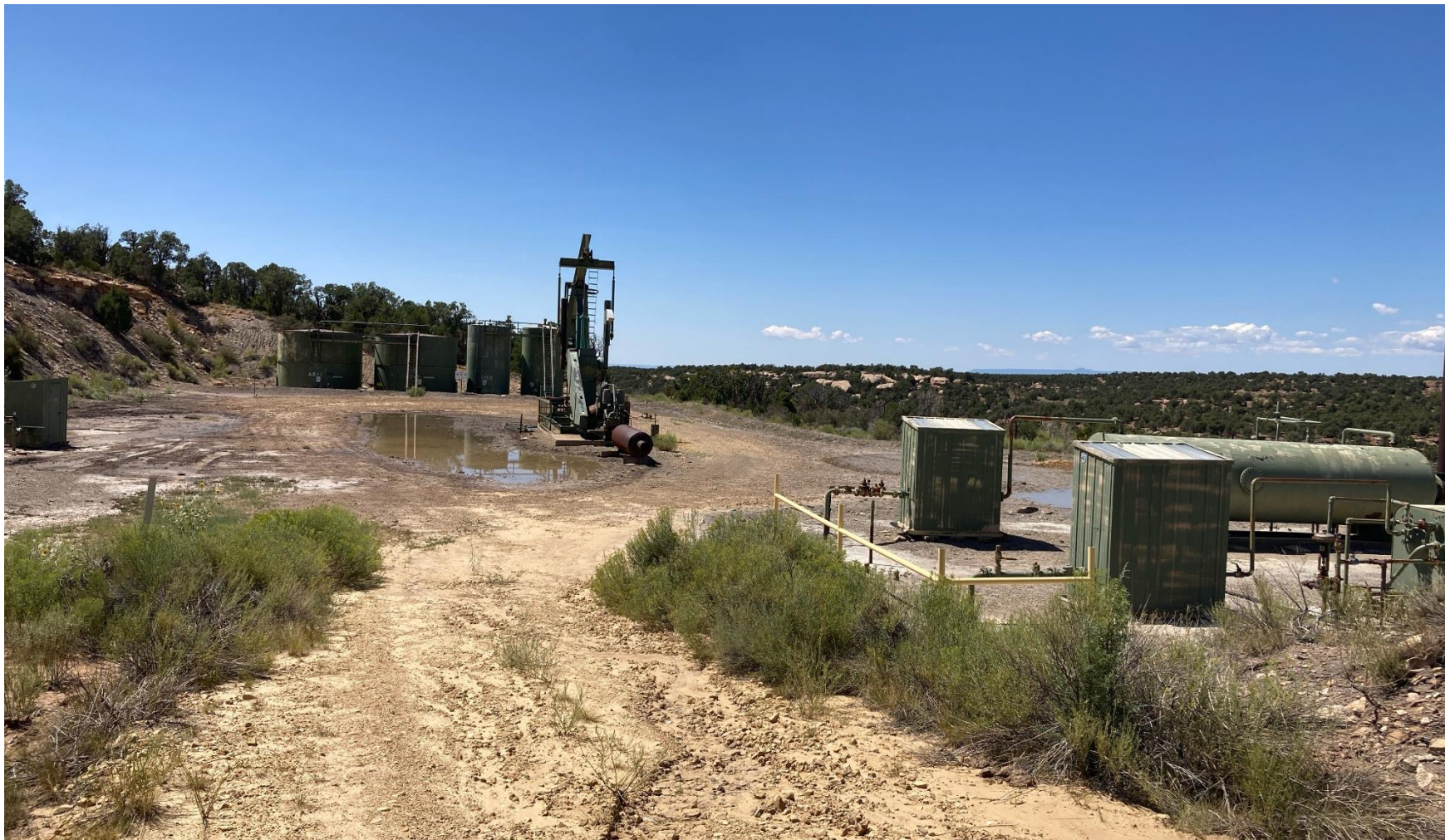
PHOTO 2: LOCATION/ STORMWATER POOLING IN THE MIDDLE OF LOCATION NEXT TO WELLHEAD. INSTALL BMP'S TO PREVENT STORMWATER POOLING ANYWHERE ON LOCATION PER RULE 1002.
