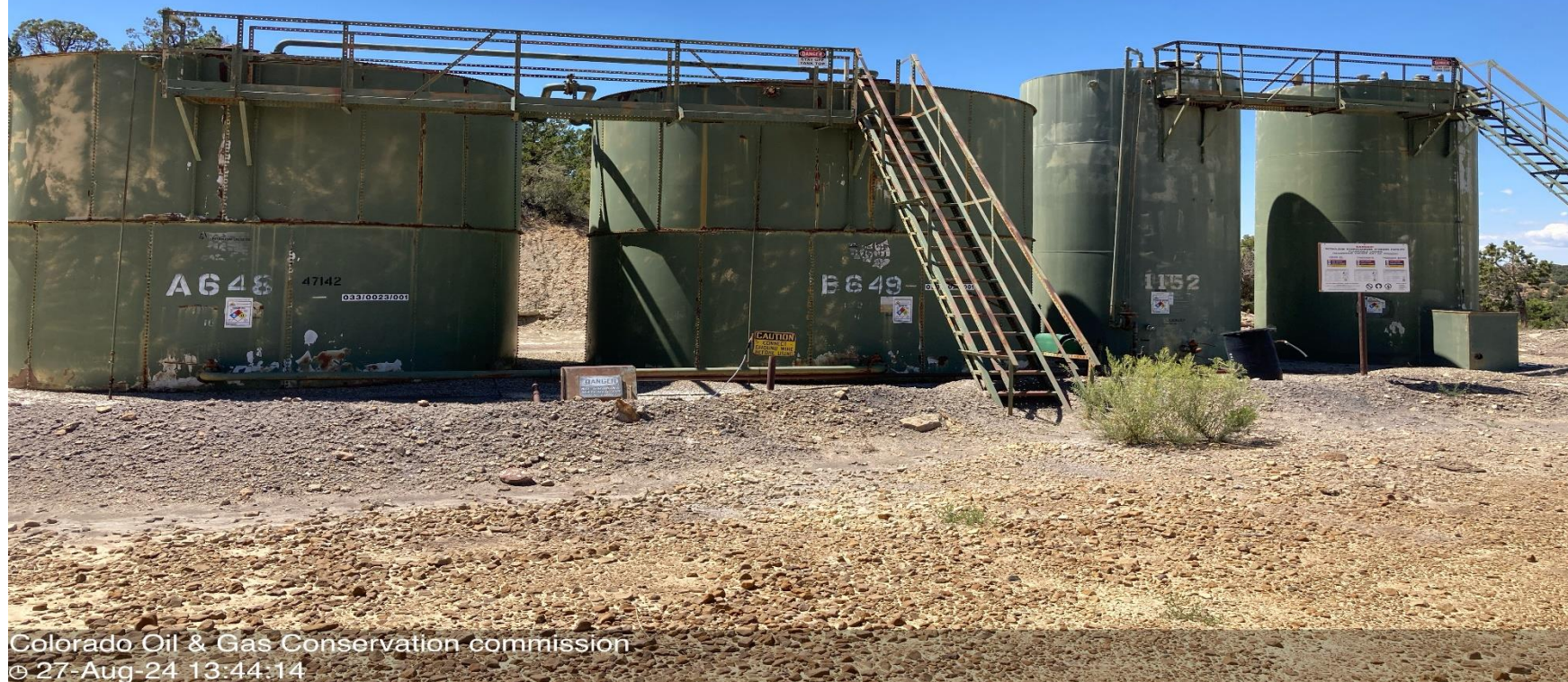
PHOTO 4: CRUDE OIL AND PRODUCED WATER TAK BATTERY.
