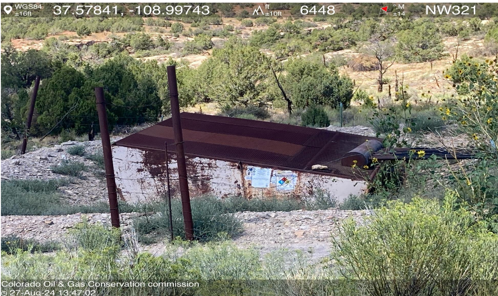
PHOTO 5: OPEN TOP PRODUCED WATER TANK BATTERY.
