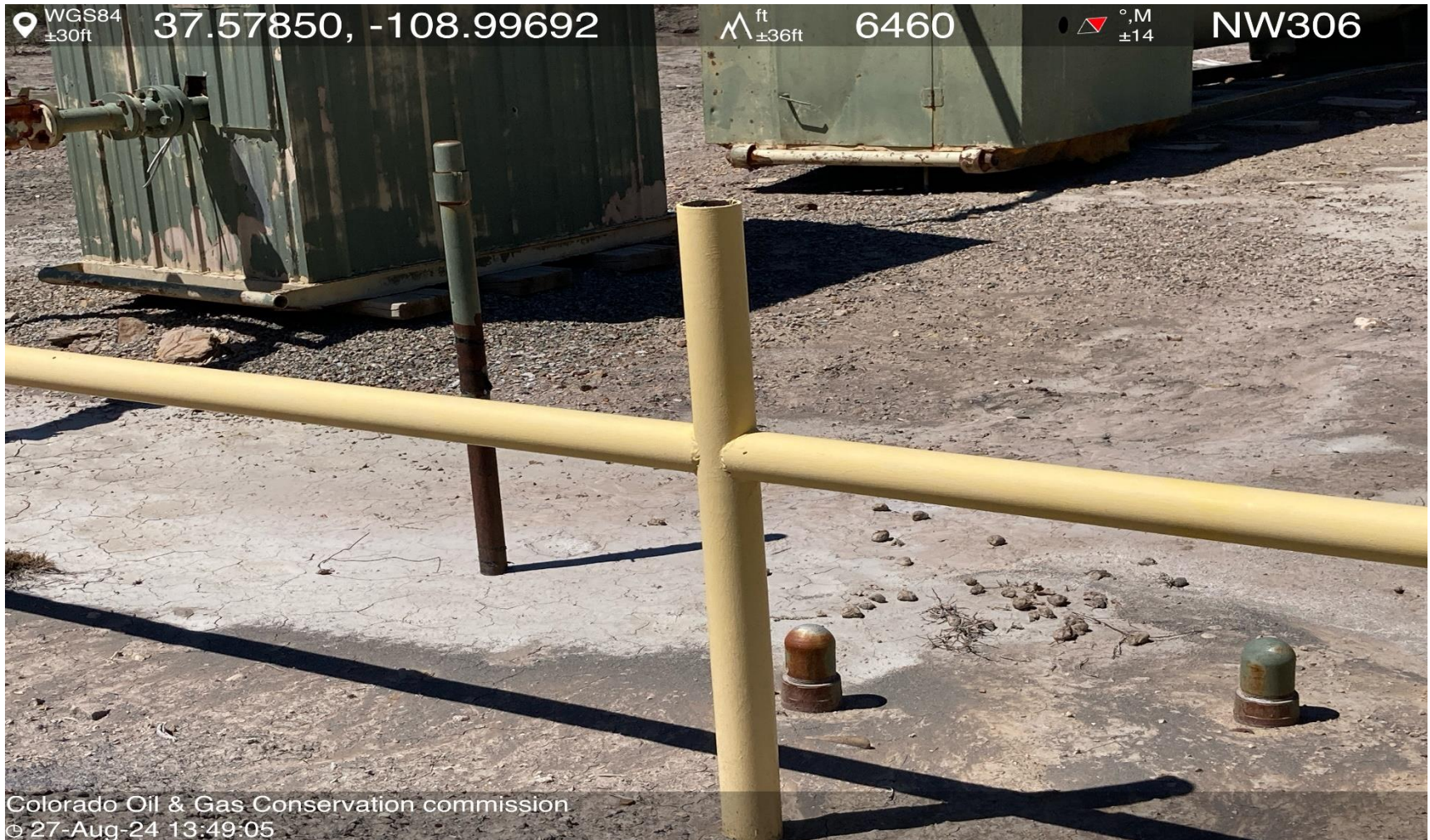
PHOTO 11: UNUSED EQUIPMENT (2 3" RISERS AND 1 2" RISER NEAR HEATED SEPARATOR). REMOVE OR MARK RISERS FOR WHAT THEY CARRY (IE. WATER, GAS ECT.). PER RULE 606.
