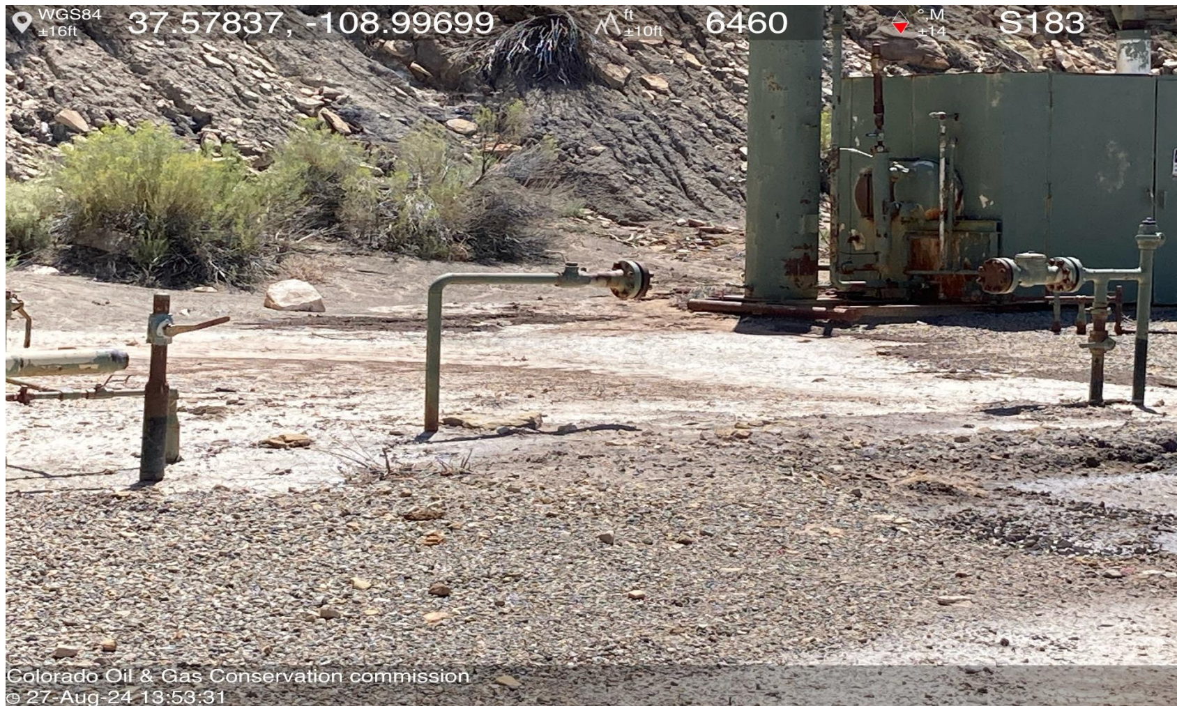
PHOTO 8: UNUSED EQUIPMENT (3 2" RISERS NEAR COMPRESSOR). REMOVE OR MARK RISERS FOR WHAT THEY CARRY (IE. WATER, GAS ECT.). PER RULE 606.
