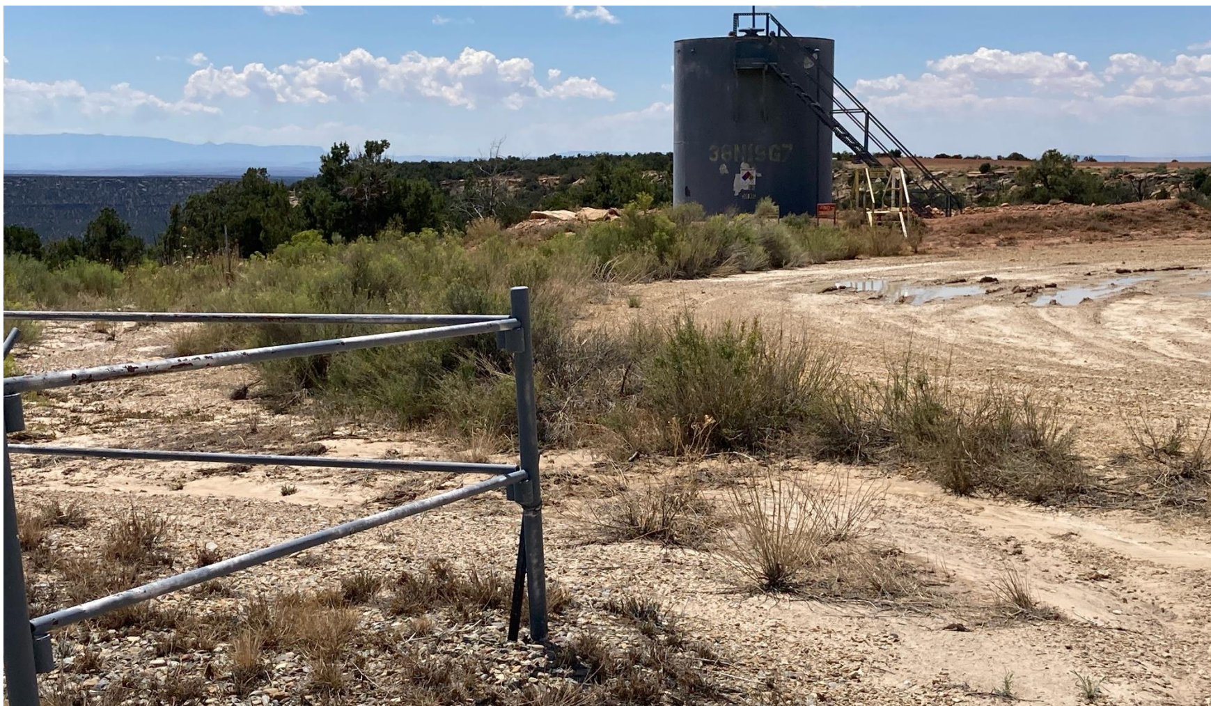
PHOTO 8: WEEDS AROUND LOCATION ARE NOT MAINTAINED. MAINTAIN WEEDS AROUND LOCATION, REMOVE WEEDS INSIDE SECONDARY CONTAINMENT BERMS PER RULE 606,
