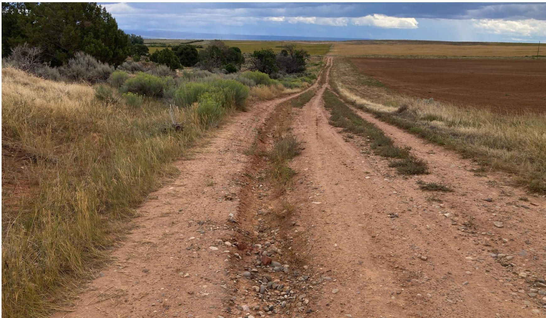
PHOTO 5: VEHICLE TRACKING AND STORM WATER HAVE ERODED ROW AND IS CAUSING VEHICLE TO SIDETRACK AND MAKE ROAD WIDER. REPAIR ROW AND INSTALL BMP'S TO PREVENT VEHICLE TRACKING AND STORMWATER EROSION PER RULE 1002.
