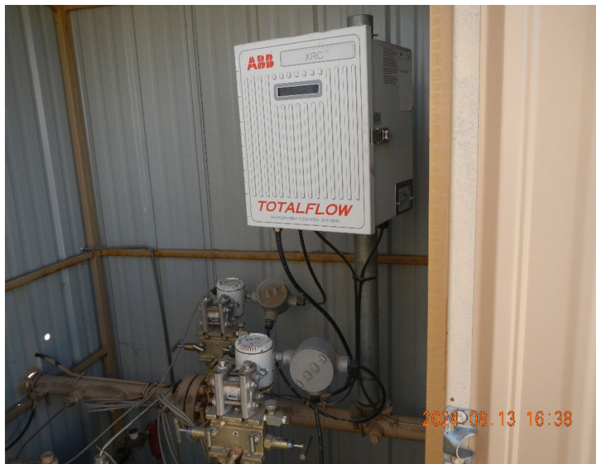
5. Digital meter inside remote meter shed.
